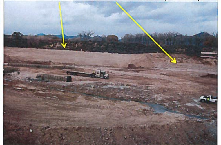
View from the south side of Mine Cell B, facing north. Much of the north slope of the pit has been graded to 3H:1V or less. The active mine face is shown on right side of the photo.
