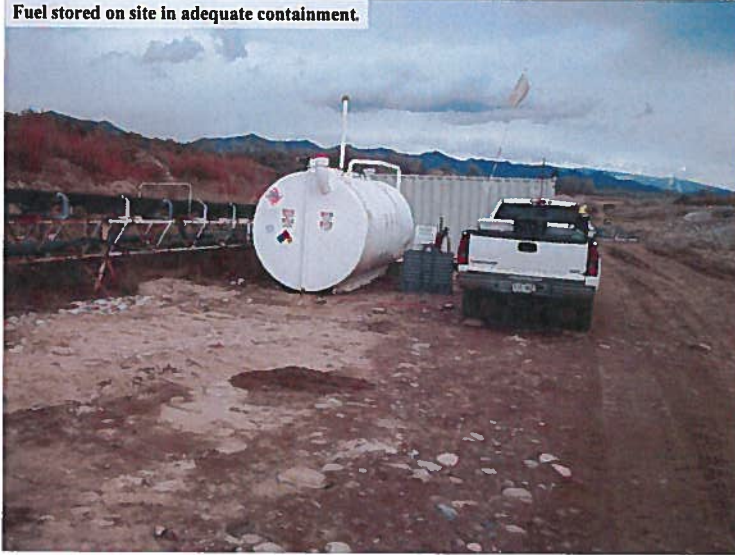
Fuel stored on site in adequate containment.
