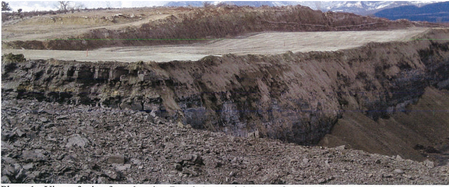
Photo 1: View of mine face showing Bench 1 material (upper face) and lower overburden material.
