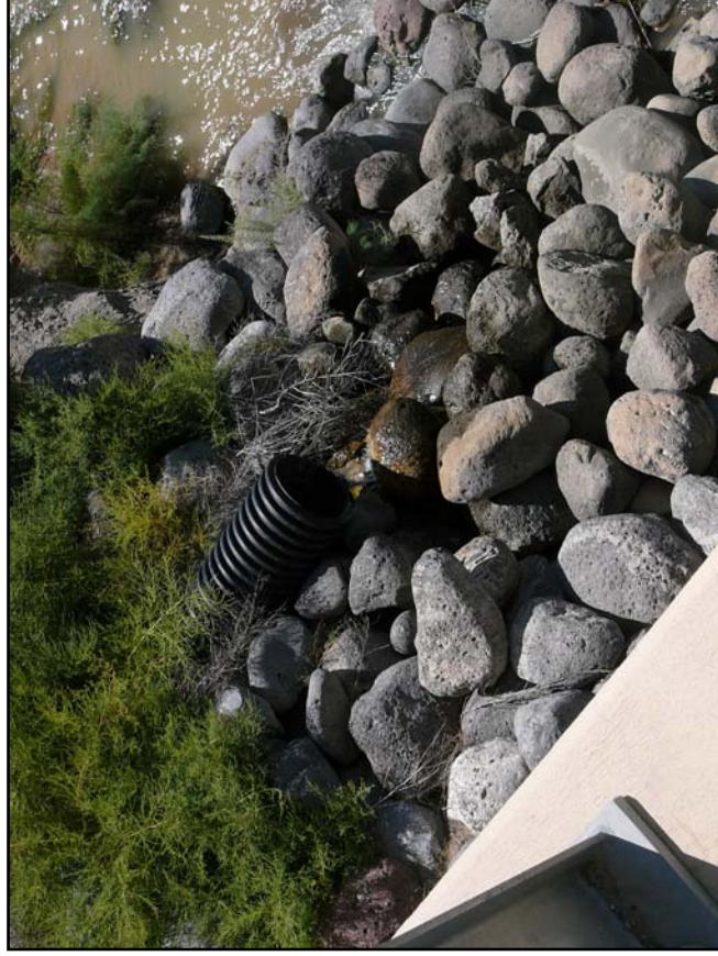
Photo 10. West end of concrete ditch in polygon S, most of the water has leaked into the borrow ditch by this point
