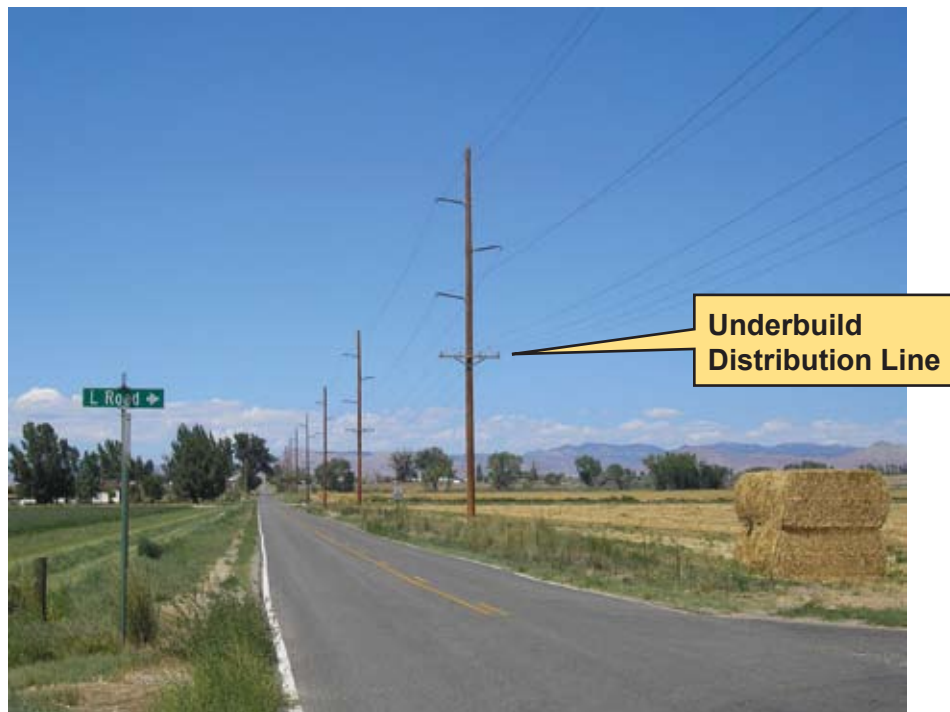
Typical Transmission Pole and Conductors with Underbuild Distribution Line
