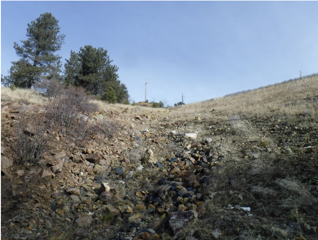
Photo 7: Another photo where dam placed material (right side of photo) meets native material (left side of photo)
