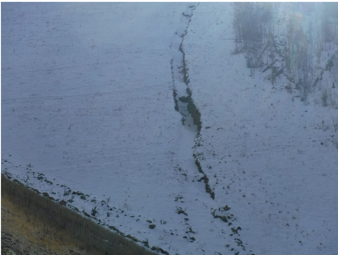
Photo 8: Deep erosion feature on the other side of the dam, zoomed in
