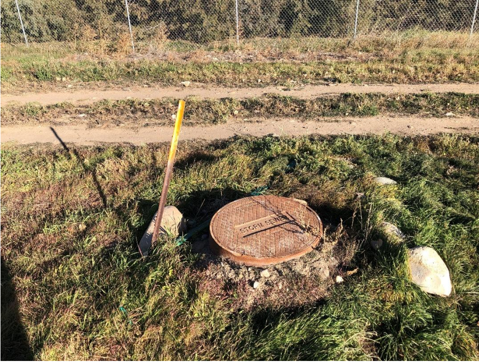
Photo 5. West pond, east side – manhole cover for underdrain
