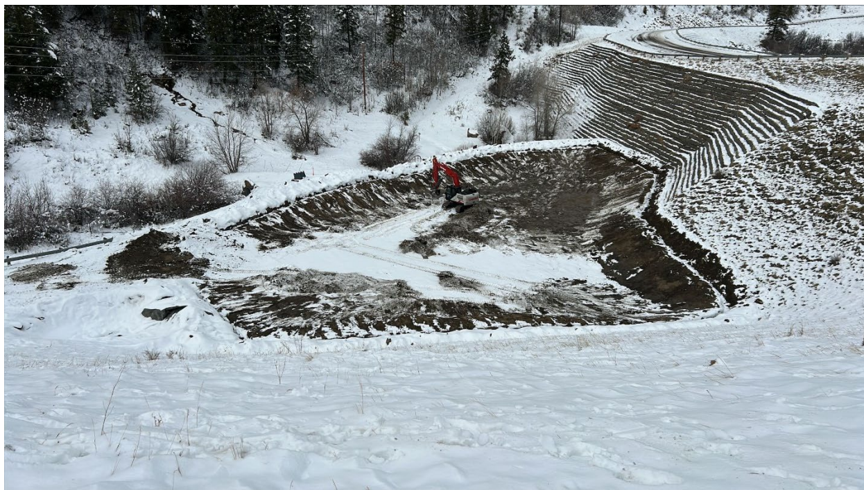
Figure 6: SG-1 pond, being prepared for installation of new liner
