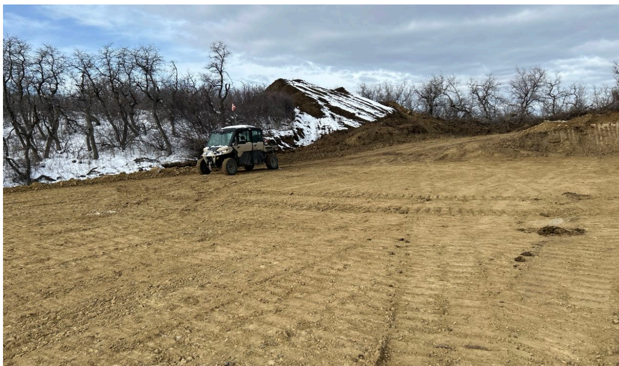
Figure 18: B26-4 pad level and compacted
