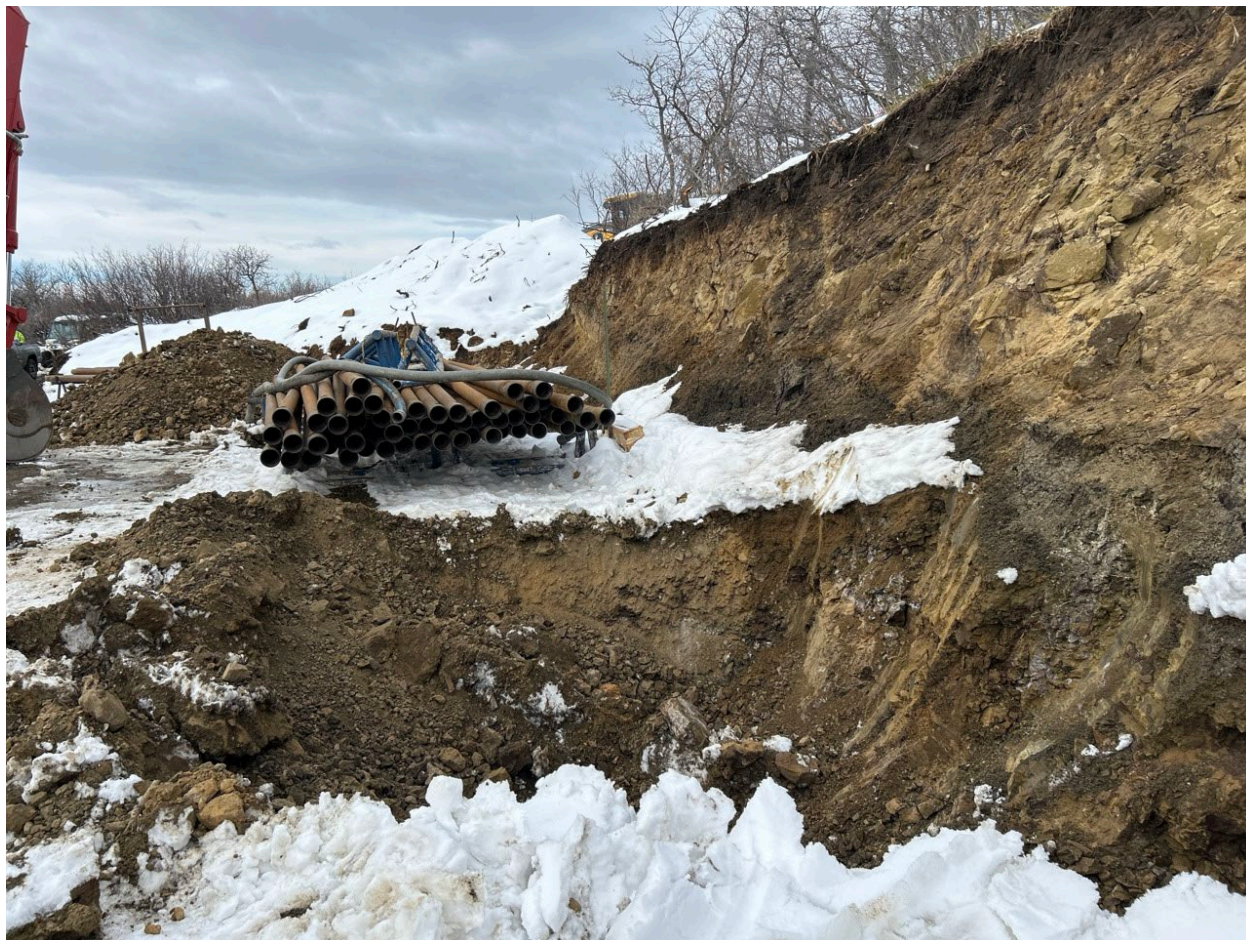
Figure 13: Second mud pit on B26-2 under construction
