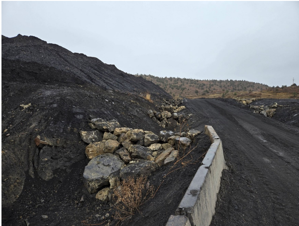
Photo 25: Looking east at the repaired check dams on both sides of the RDA haul road.
