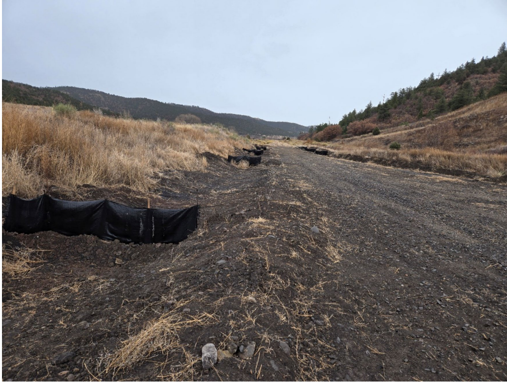
Photo 11: Looking east at the silt fences in the S.A.E on the south side of Pond 007A on the northside of the access road.
