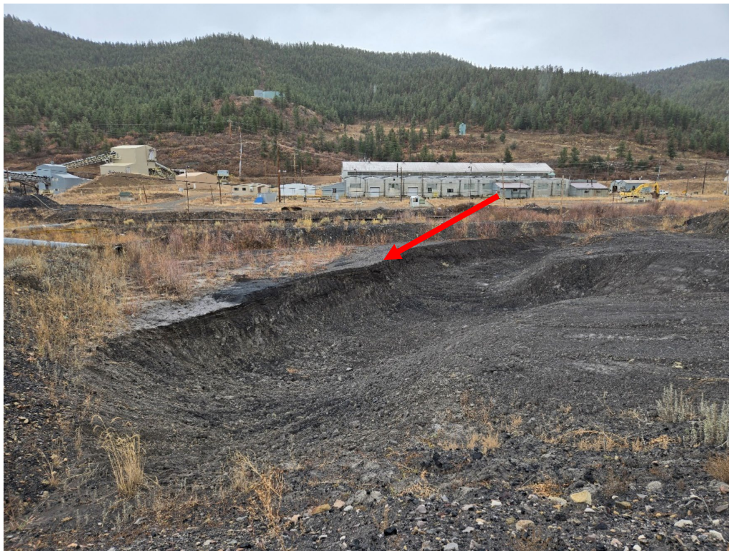
Photo 1: Looking south at the excavated sediment basin on the east end of DWDA #2. The arrow points to the previous floor height of the sediment basin.
