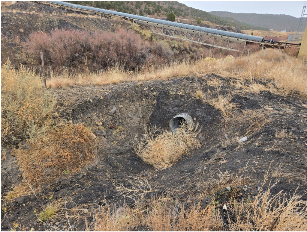
Photo 14: Looking northeast at where the erosion in ditch D34 was repaired and at the cleaned-out inlet side of C64.
