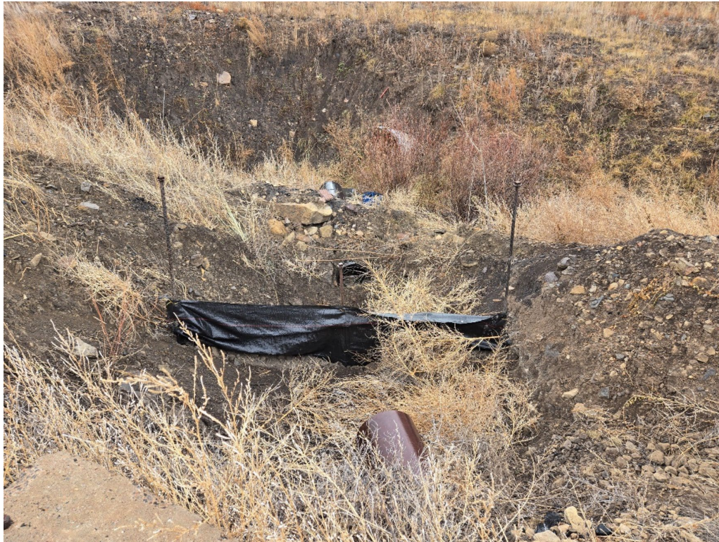
Photo 13: Looking south at the repaired silt fence near culvert C90.
