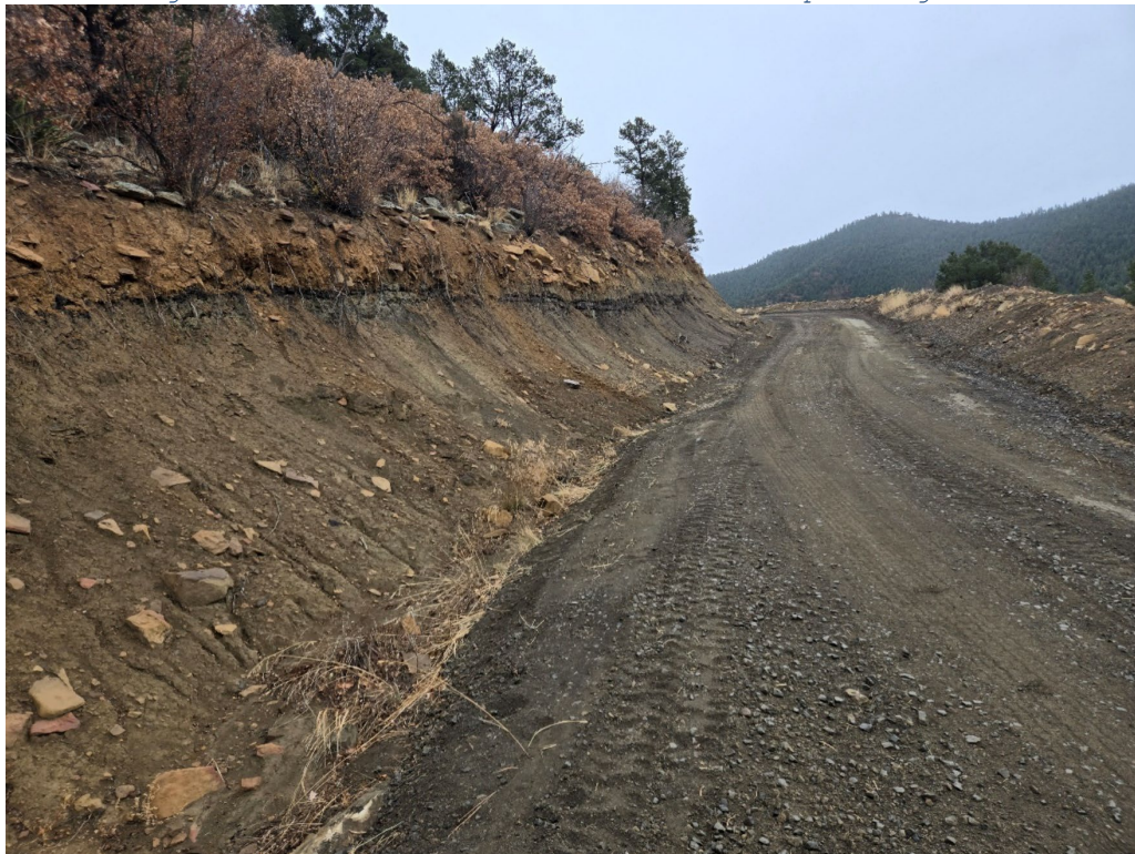
Photo 28: Looking east along the regraded haul road where falling rocks have been removed and
