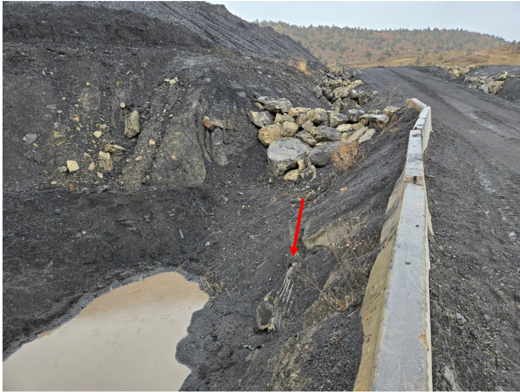
Photo 23: Looking east at the cleaned-out sediment sump in front of the C81 inlet (arrow).
