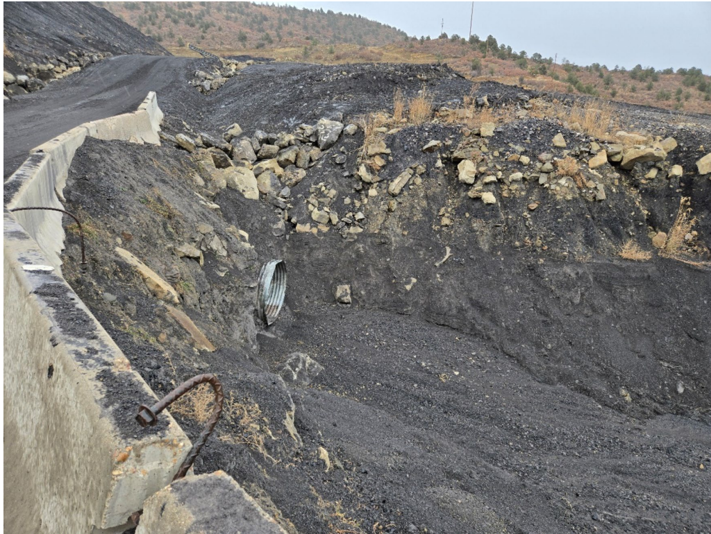
Photo 24: Looking east at the cleaned-out sediment sump in front of the C81 outlet.
