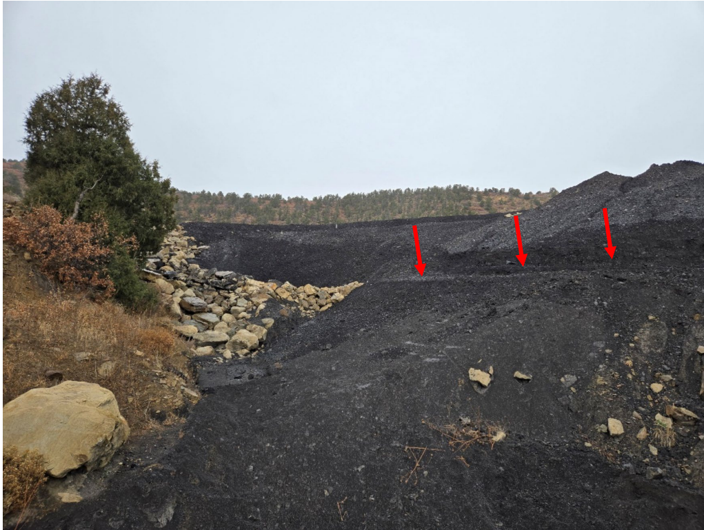
Photo 21: Looking northwest at the repaired erosion on the west side of the RDA. The arrow points to where the Operator created a temporary road to conduct maintenance in this area.
