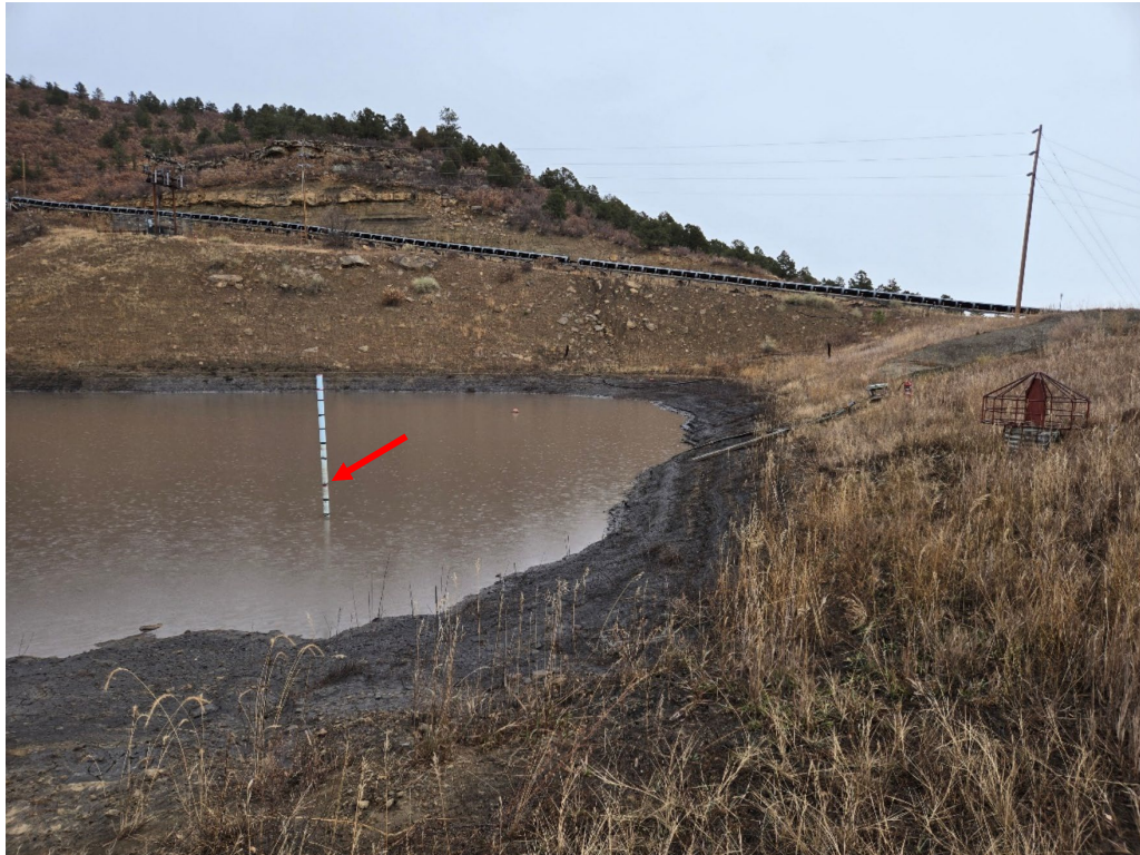
Photo 7: Pumping the water to Ponds 6 and 7 lowered the water level by 4 or 5 feet in Pond 08. The arrow points to maximum capacity level maintained when the site was operating.
