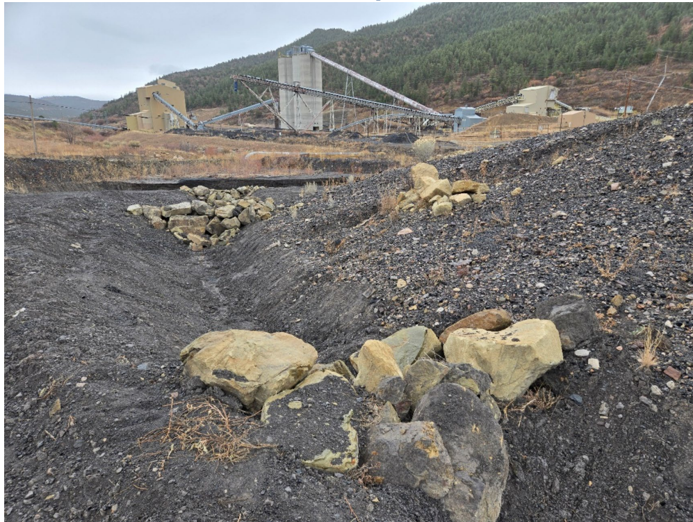
Photo 3: Looking east at the cleaned and repaired check dams within D12 leading to the sediment basin on the east side of DWDA #2.
