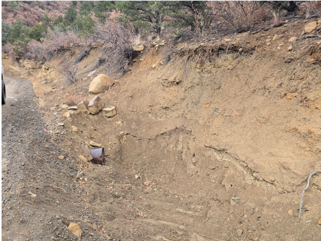
Photo 27: Looking at one of the cleaned-out sediment sumps along the RDA haul road.
