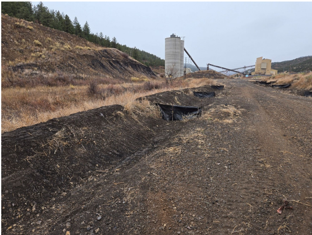
Photo 12: Looking west at the silt fences in the S.A.E on the south side of Pond 007A on the
