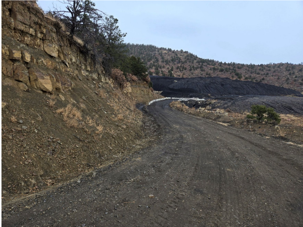
Photo 26: Looking north at the cleaned-out Ditch D56 alongside the haul road, where fine grey sediment had previously been deposited onto the road.
