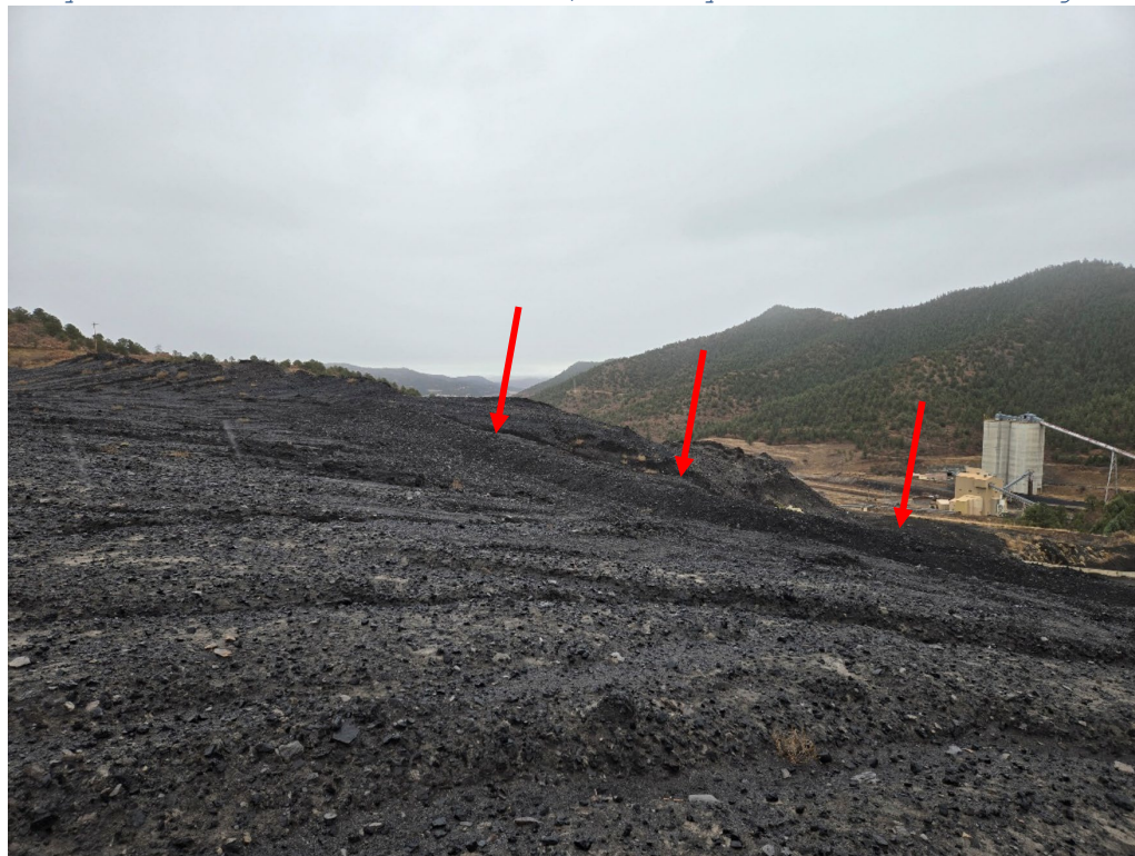
Photo 22: Standing on top of the RDA looking at the new berm along the top that will help divert stormwater runoff straight to the armored channel in Ditch D55.
