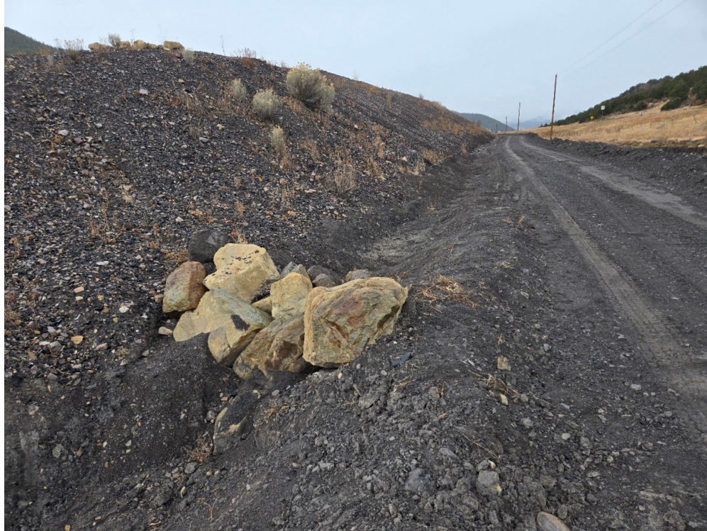
Photo 2: Looking west at Ditch D12 on the north side of DWDA #2. The check dams within D12 have been repaired.
