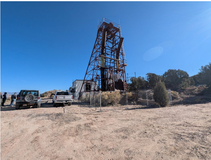
Head frame and hoist/compressor structures remain on site. Temporary fencing installed.
