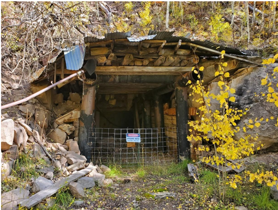
Photo 2: View to the east of the portal.
