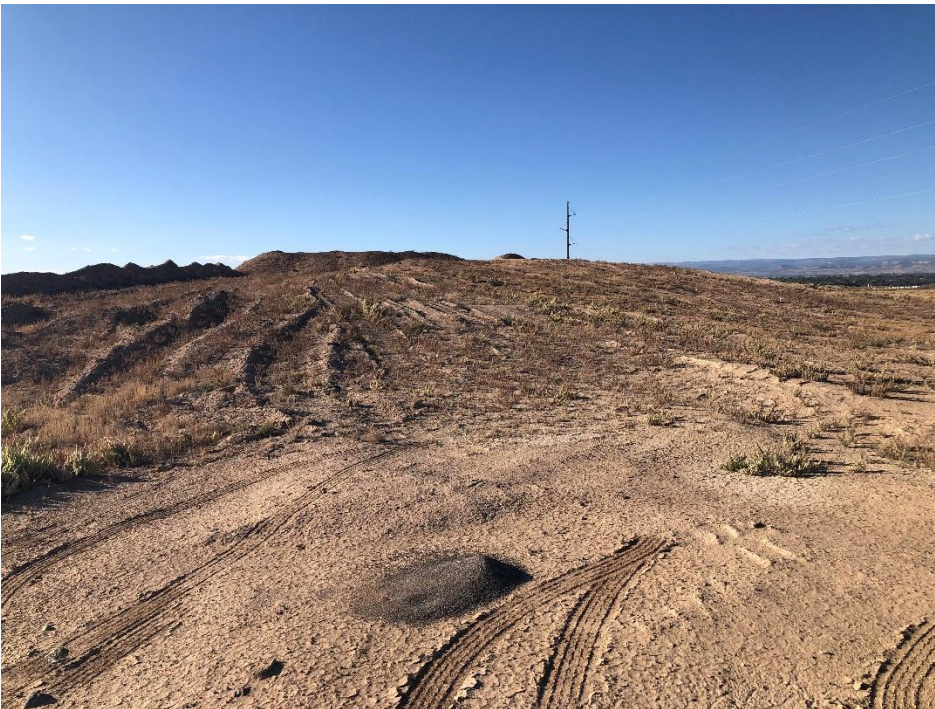
Photo 8. Topsoil stockpile with some vegetation (erosion BMPs are recommended)
