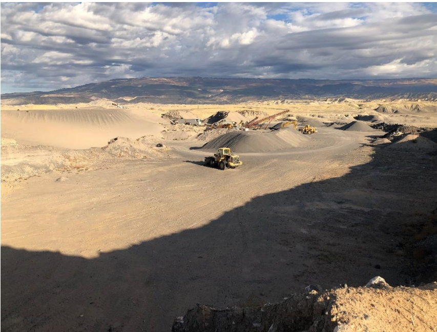
Photo 2. Processing area and stockpiles
