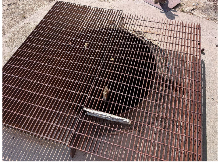
Vent shaft secured with steel grating welded to collar
