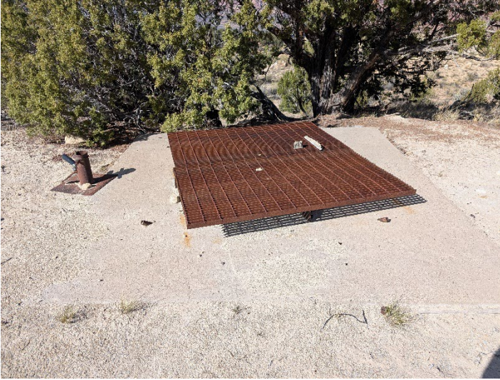
Vent shaft secured with steel grating welded to collar
