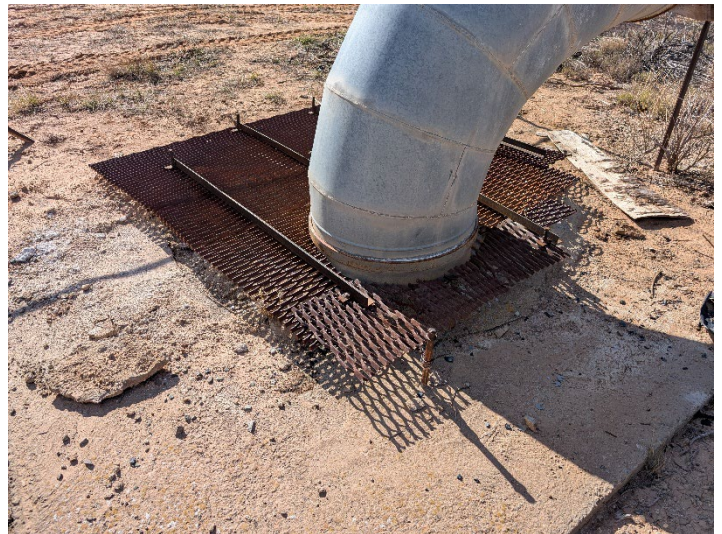
Ventilation fan shaft – fan removed, shaft not yet secured
