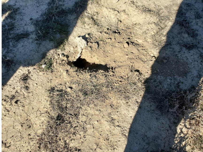
Photo 9: View to the north of animal burrow on the RP-5 Pond embankment.
