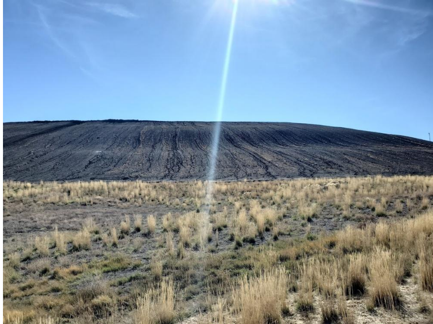
Photo 11: View to the south of rills on the RP-2/3/4 Pile
