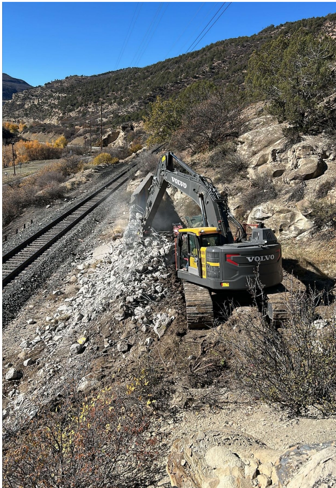
Figure 17: Demolition of Pond C embankment
