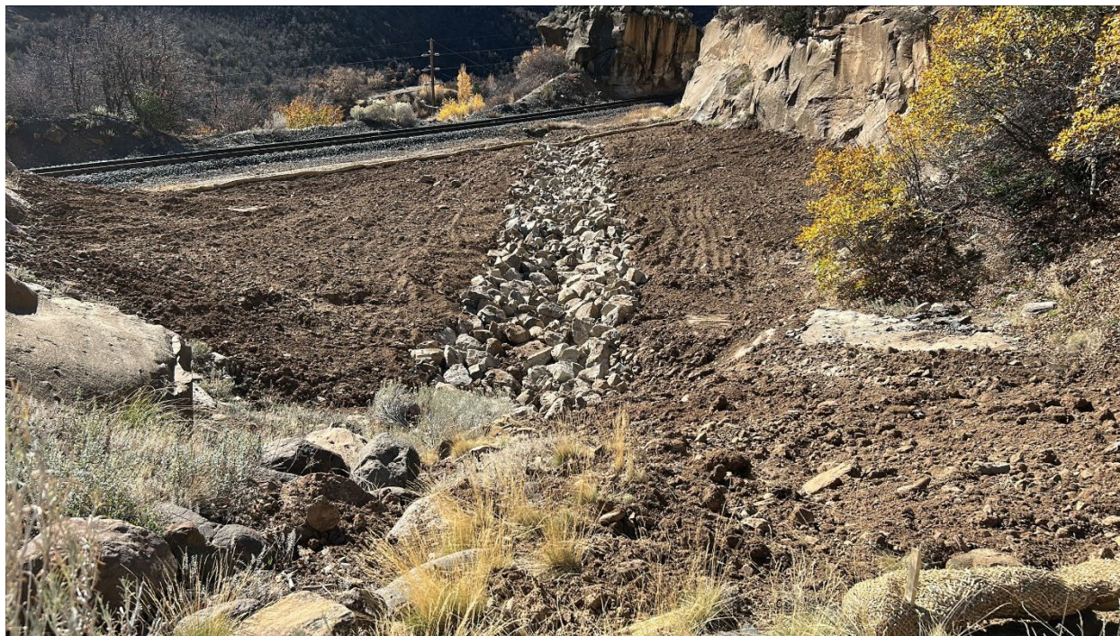
Figure 10: Extension of armored drain
