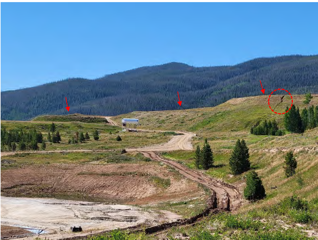
Photo 16: Looking southwest at the three benches of the North Topsoil Stockpile Area. Erosional rill observed on the top bench noted by red circle.
