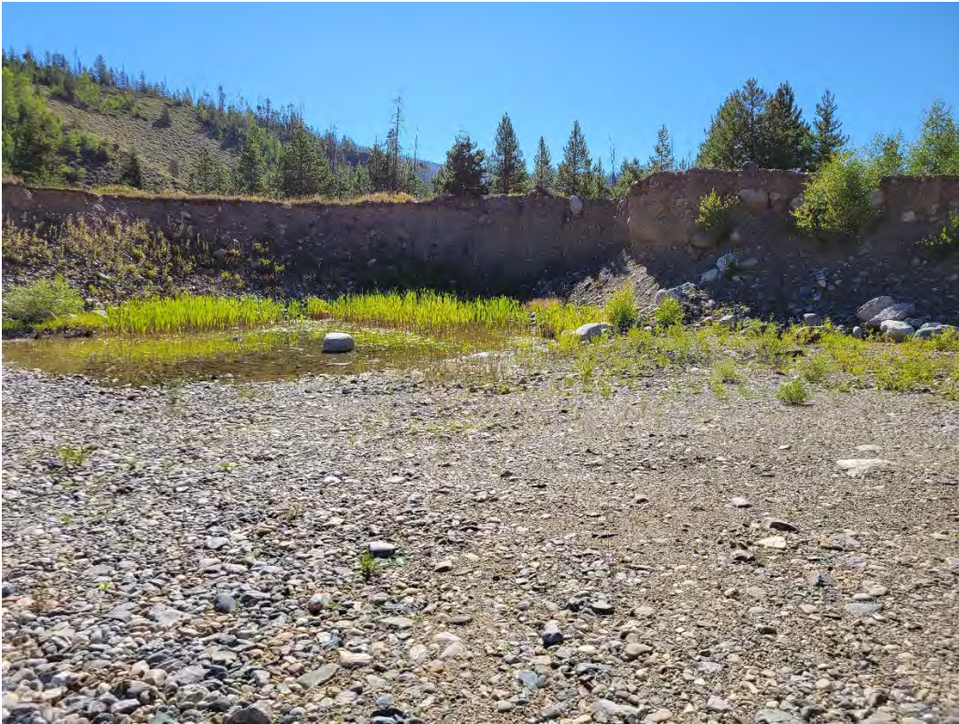
Photo 5: Standing water observed at the base of the highwall on the east side of the pit.
