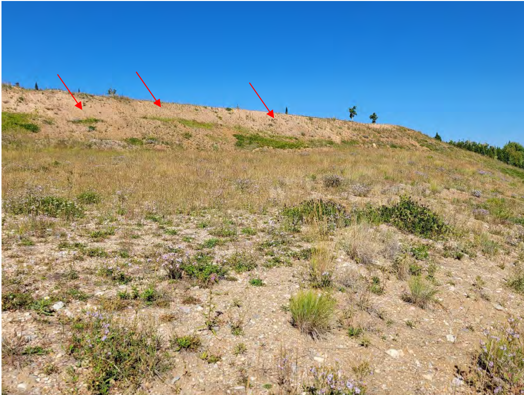
Photo 19: Looking at the east side of the top bench in the North Topsoil Stockpile area. Slope steeper than 3H:1V noted by red arrows.
