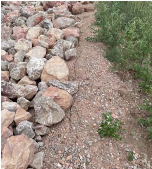
8. SETTLEMENT CRACKS ON EDGE OF BENCH.
