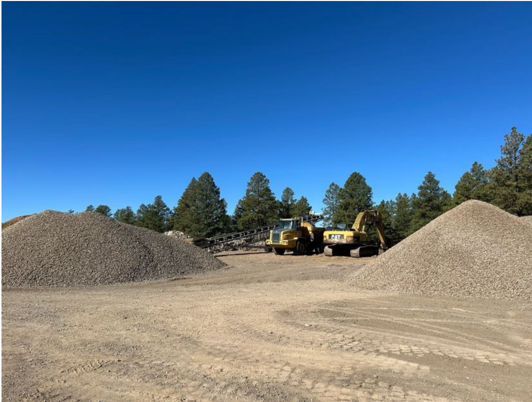
Photo 9: View of stockpiles of mined material and equipment within the Phase 3 area, facing west.
