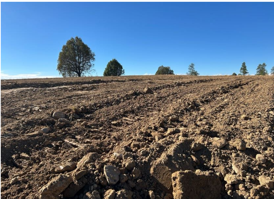
Photo 8: View of spread topsoil within the Phase 3 area, facing south.
