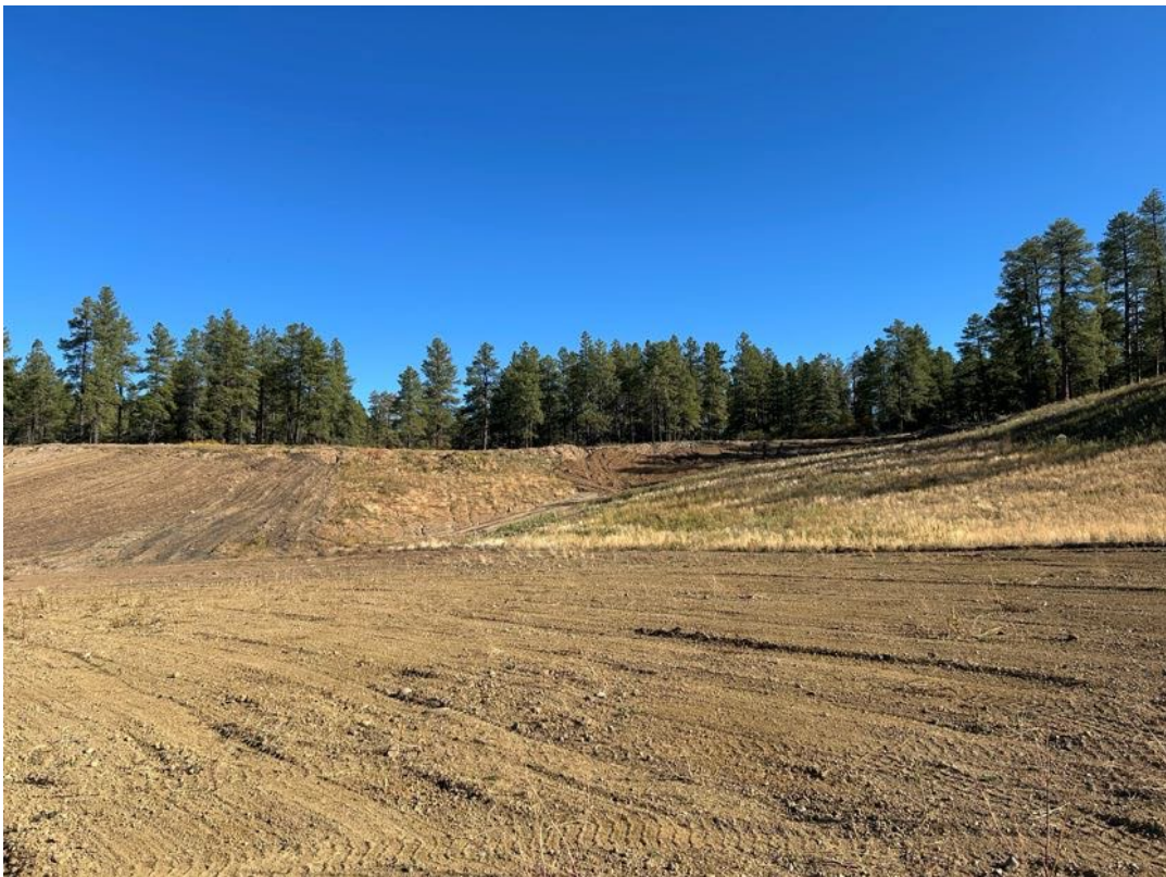
Photo 4: View of the graded pit slope at a 3:1 configuration, facing north.
