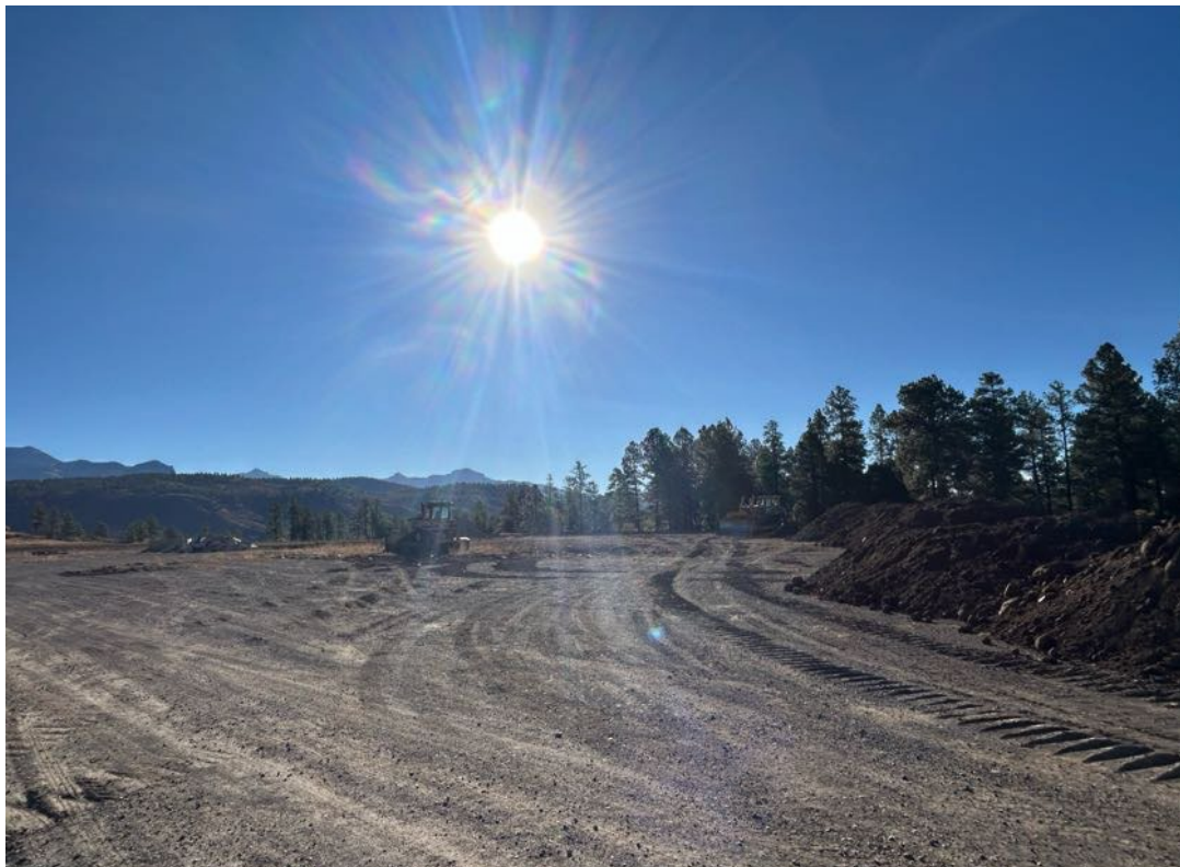
Photo 2: View of Phase 1 and 2 area, two bulldozer, and the spreading of topsoil. Facing east.
