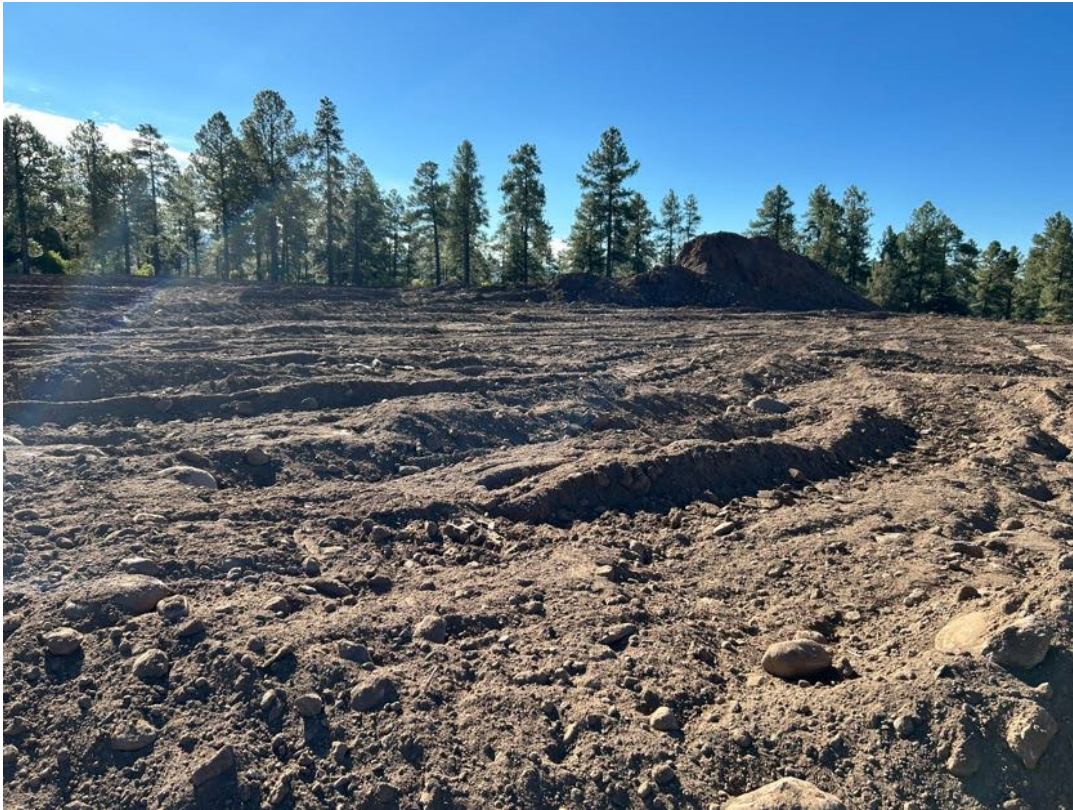
Photo 3: View of a topsoil stockpile and topsoil being spread in the Phase 1 and 2 areas, facing south.
