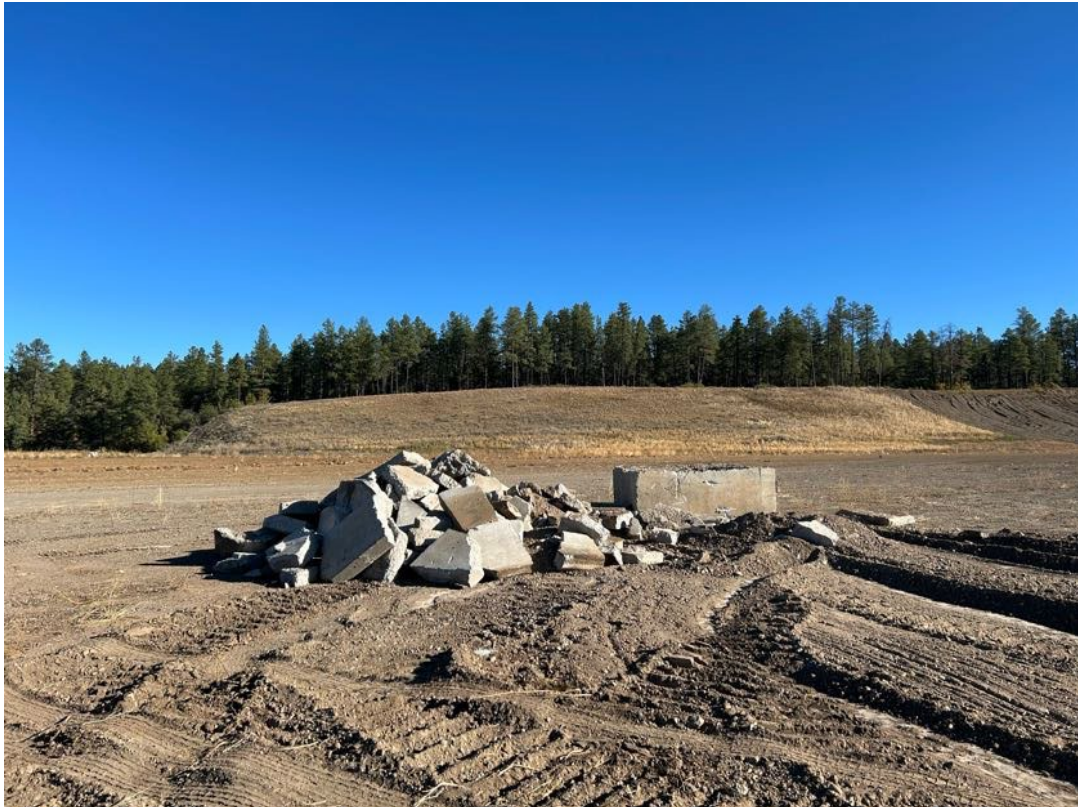
Photo 7: View of a pile of concrete, as well as the portion of the pit slope that has been revegetated facing north.
