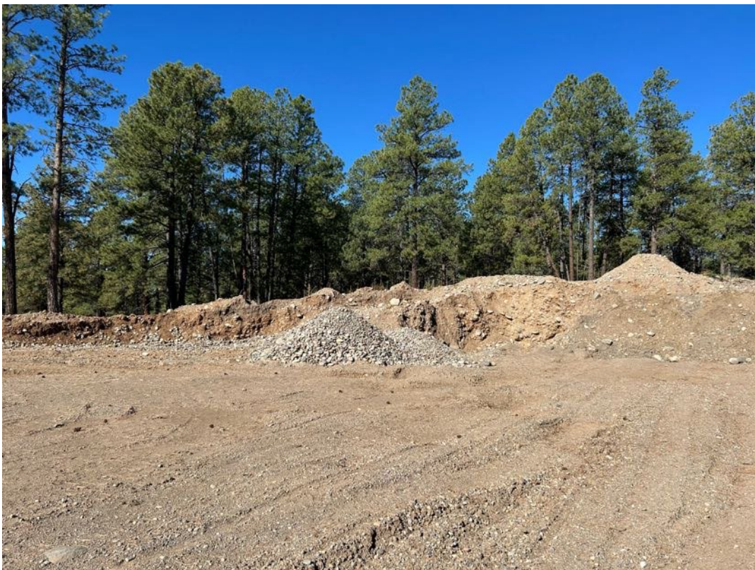
Photo 10: View of a stockpiled material on the north edge of the affected area boundary within the Phase 3 area, facing west.
