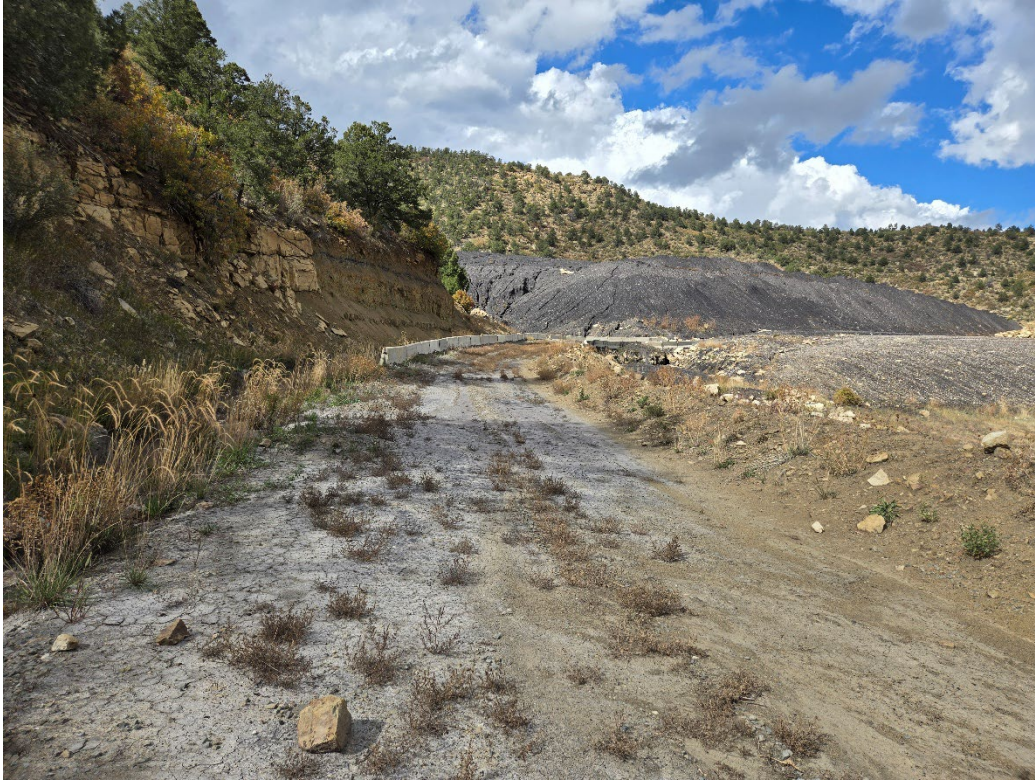
Photo 24: Looking north at the fine-grained grey material deposited on the road from ditch D56.
