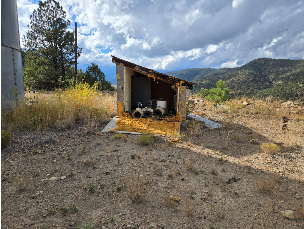
Photo 29: Damaged water pump/valve cover structure.
