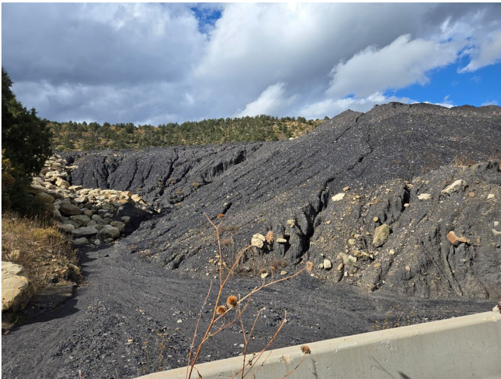
Photo 22: Looking north at the excessive erosion on the west side of the RDA slopes.
