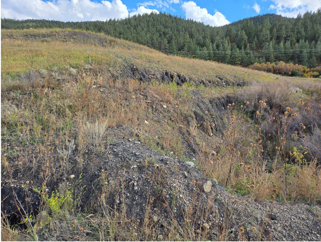
Photo 27: Looking southeast at the berm dividing the clean diverted surface water (D7) from the water contacting disturbed areas (ditch that discharges into D6). The right side has bindweed growth.
