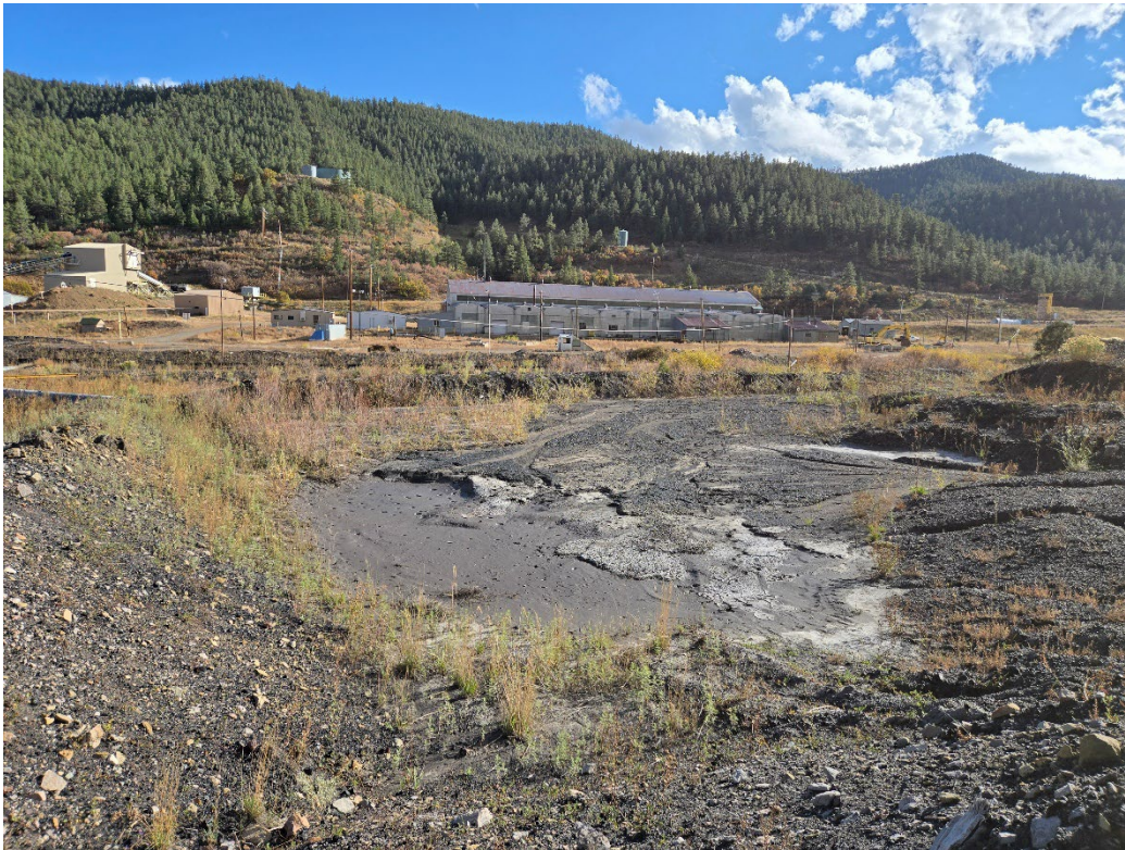
Photo 3: Sediment basin on east side of DWDA #2.
