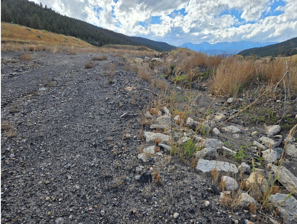
Photo 18: Check dams within the soil storage area.
