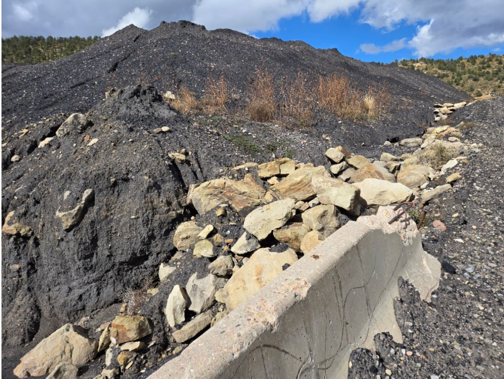
Photo 21. Looking at the damaged and eroded check dams within the ditches that lead to the inlet area for culvert C81.
