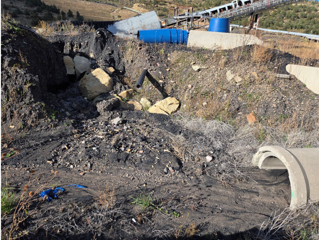
Photo 17: Check dam above C17 needs to be repaired and C17 needs to be cleaned out.
