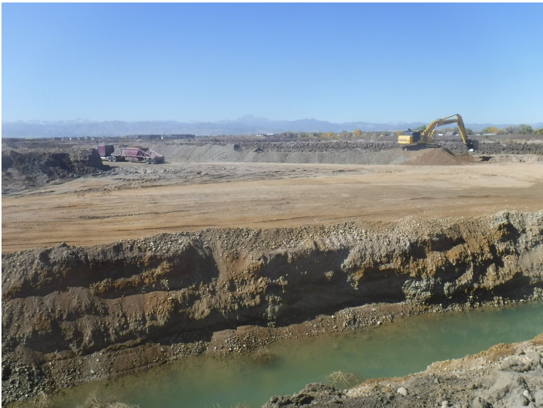
Photo 2: Mining occurring in the NE portion of Cell 4, dewatering trench in foreground
