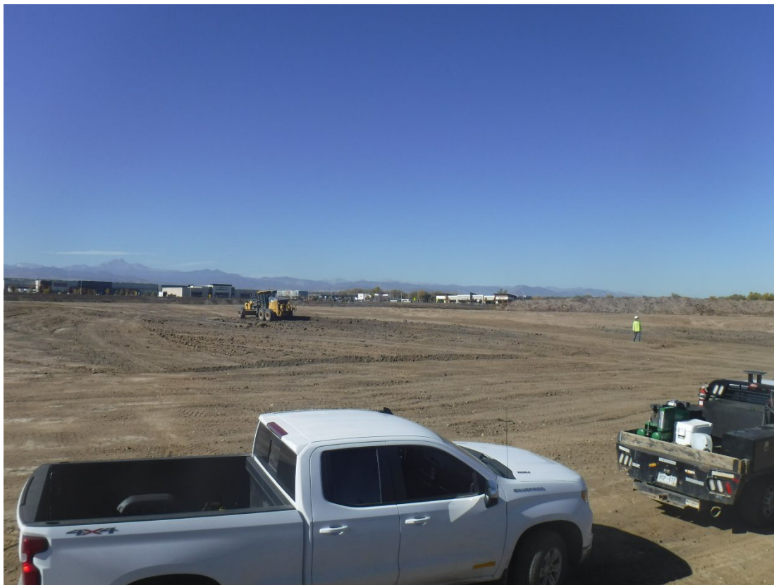
Photo 7: Backfilling and grading Cell 1
