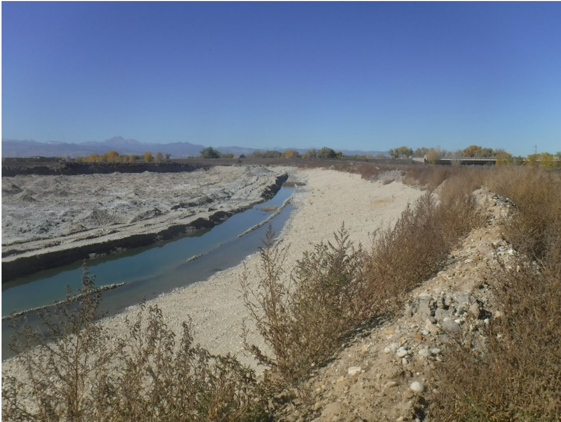
Photo 3: East side of the slurry wall that surrounds Cells 2 and 3
