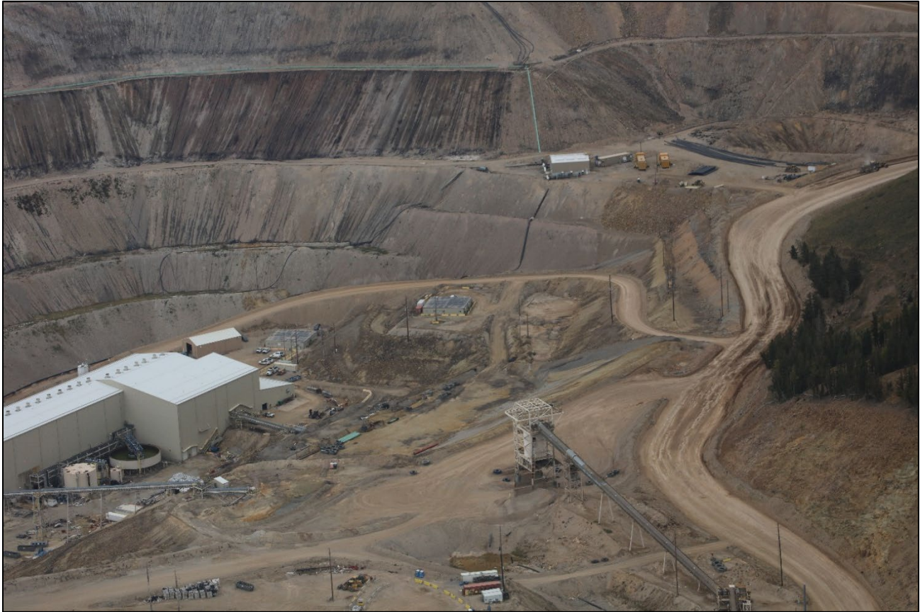
Photo 2: View north of the high-grade mill area.
