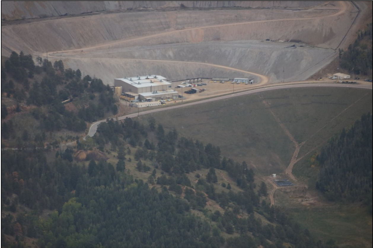
Photo 12: View north of the ADR2 facility.
