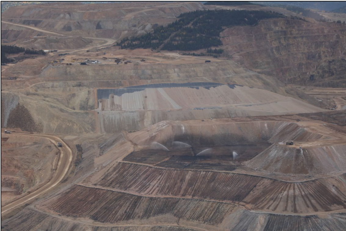
Photo 9: View east, work continues on the VLF2 Phase 3 Stage B Construction area.
