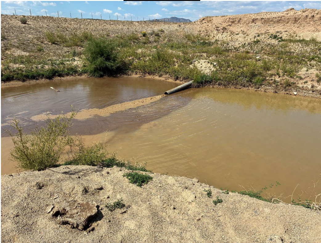
Photo 1 – Water from wash plant being pumped into sediment containment pond.
