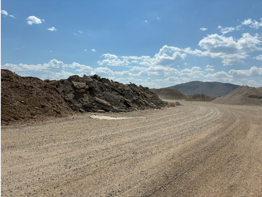
Photo 3- Recycled concrete locate by entrance road ready for processing.
