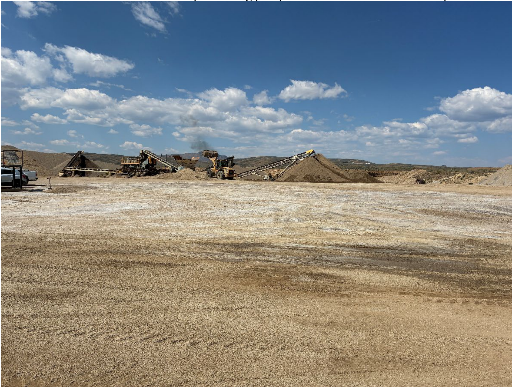
Photo 2- Wash plant in operation along with product stockpiles.
