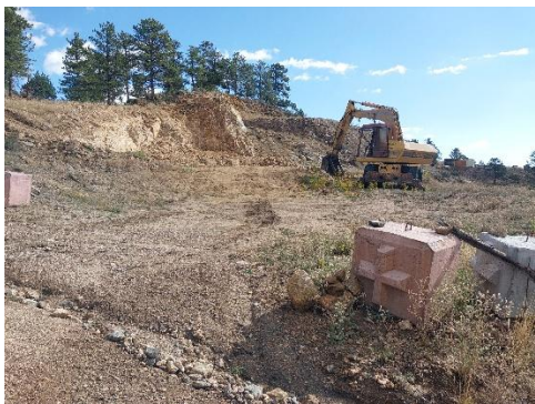
Area where work site drains to roadside ditch
