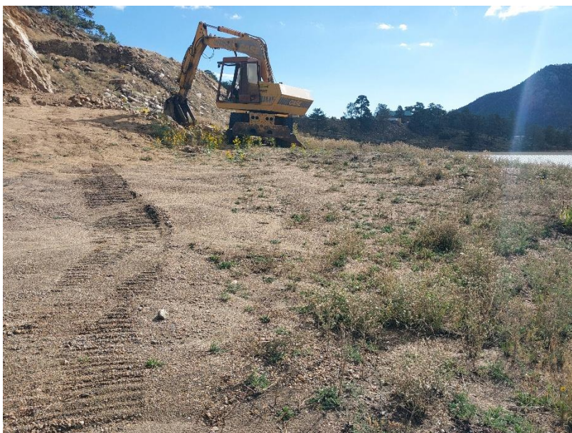
Area below wall (note lack of stockpiled material)
