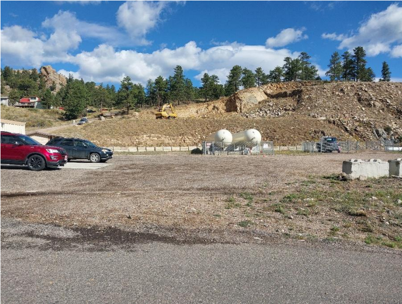
View from Kenwood Lane, south of the Polar Gas yard, looking north
