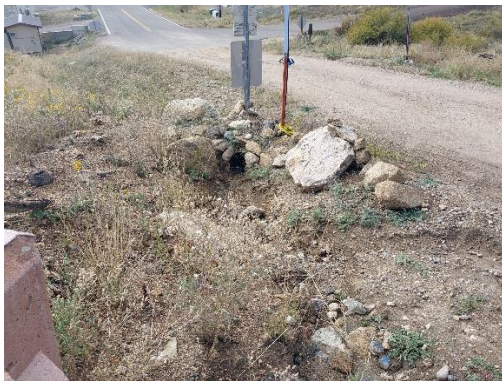
Small culvert to control runoff and prevent flooding and erosion of road
