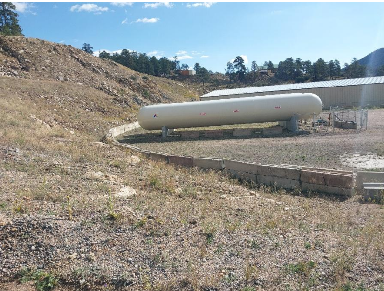
Slope between Polar Gas tanks and area in question where contractors have removed material
