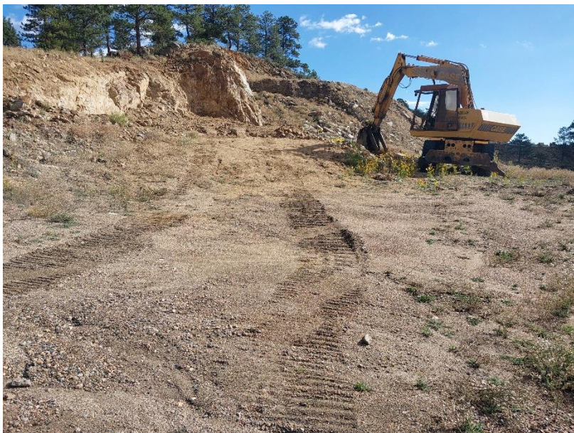
Looking east, with scrape marks apparent on wall
