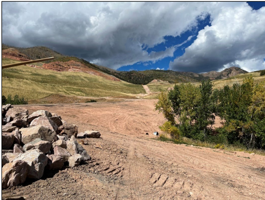
Photo 1: View west of the access road and recent drainage work.
