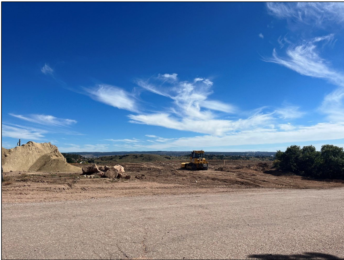
Photo 2: Grading conducted by the City of Colorado Springs for the future gravel parking lot.
