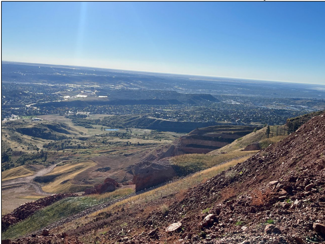
Photo 19: View southeast of the USFS drainage area and south borrow.
