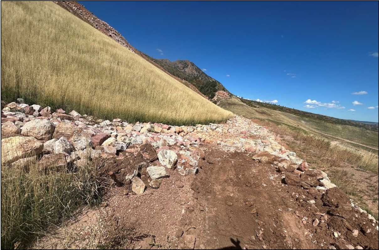
Photo 12: Sedimentation area observed at the tie in on Channels T7 and T8 has been cleaned up and the channel re-formed to direct stormwater appropriately.
