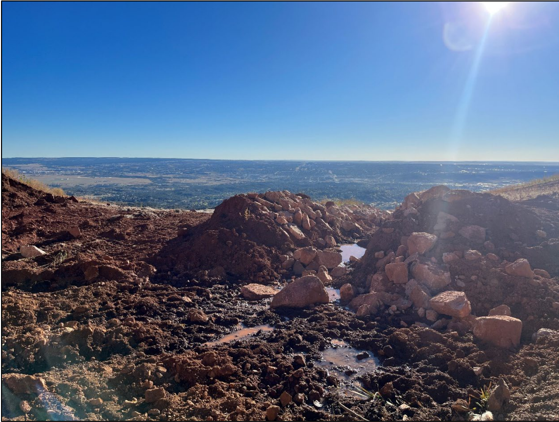
Photo 10: View east of the old 'sheep pond' area, now filled in and graded to promote drainage of natural seeps.
