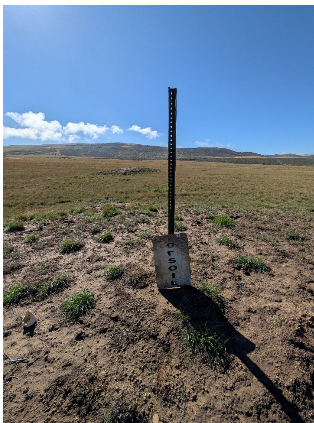
Photo 11: Topsoil pile marked with t-post and sign. Sign has fallen off the stake.
