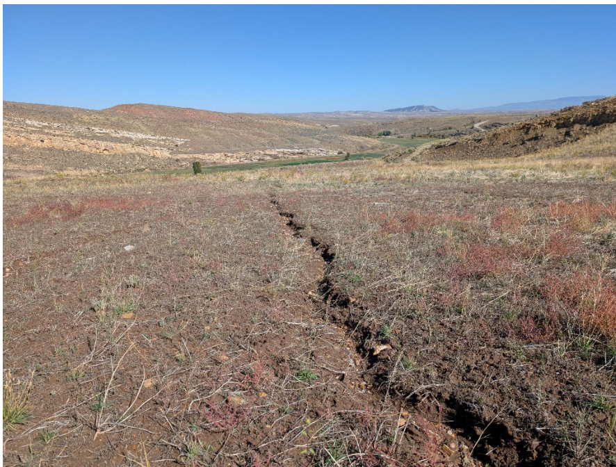
Photo 10: Erosion rill noted in slope below the #5A Portal and Service building.
