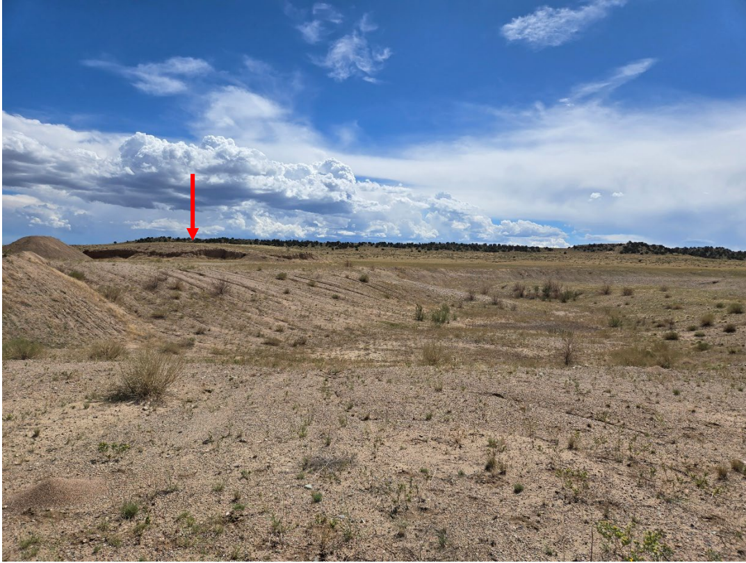
Photo 7: Looking southeast at the east and south graded slopes around the pit area. Some small erosion rills are apparent on the eastern slope. The arrow points to the topsoil pile in the background.
