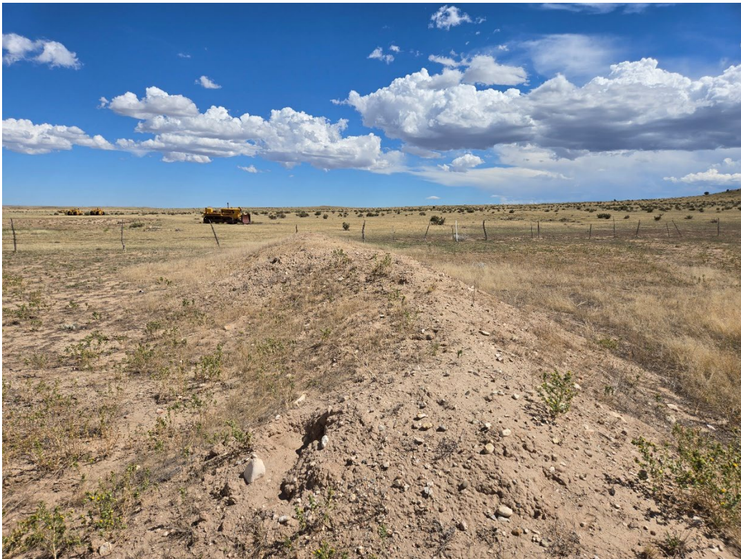
Photo 12: Looking east along the stormwater berm that marks the south side of the disturbed area.
