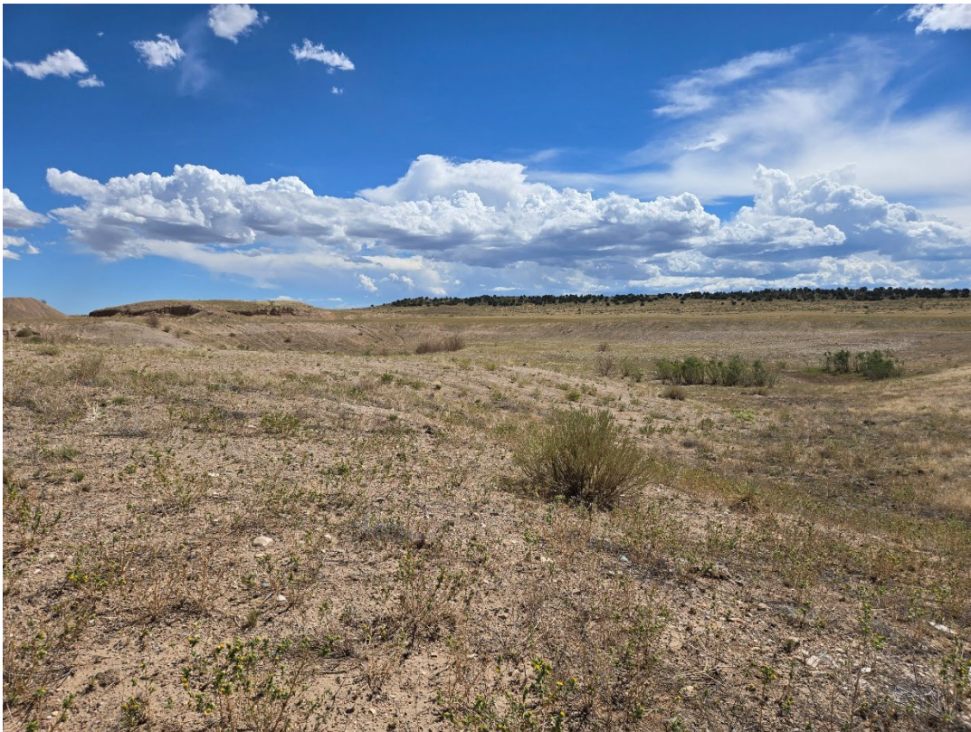
Photo 6: Looking southeast at the east and south graded slopes around the pit area. Some small erosion rills are apparent on the eastern slope.
