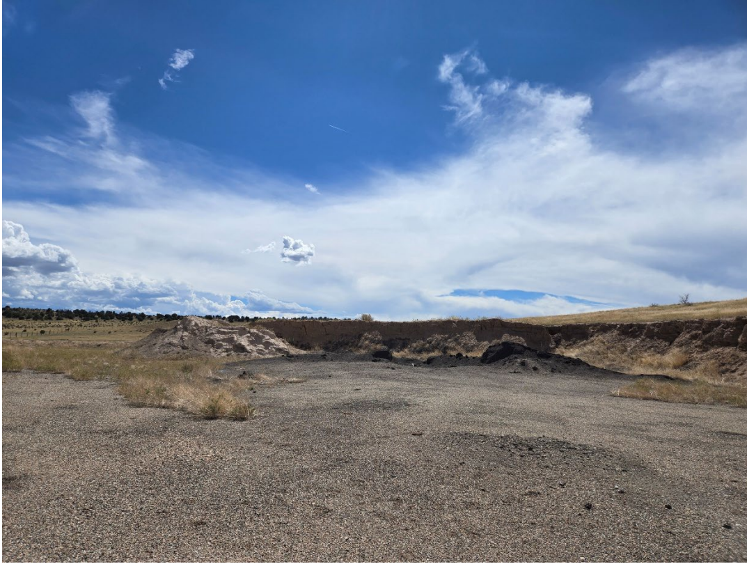
Photo 9: Looking south at a small amount of recycled asphalt, overburden, and topsoil pile on the south side of the processing area.
