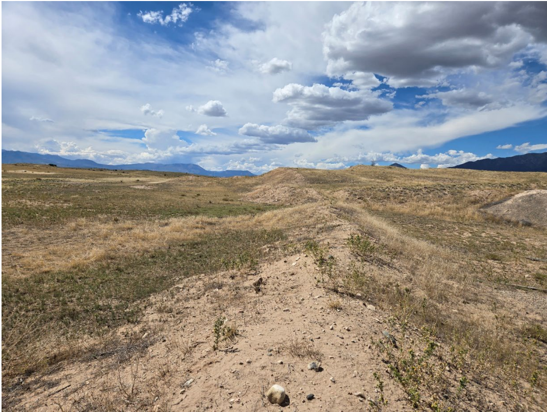
Photo 11: Looking west along the stormwater berm that marks the south side of the disturbed area.
