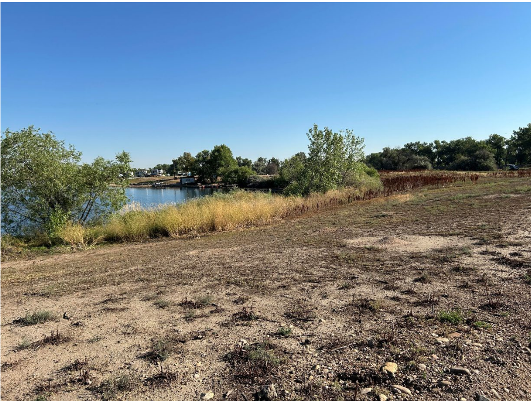
Photo 8: Mostly unsuccessful vegetation effort south of pond within Area A, facing north.
