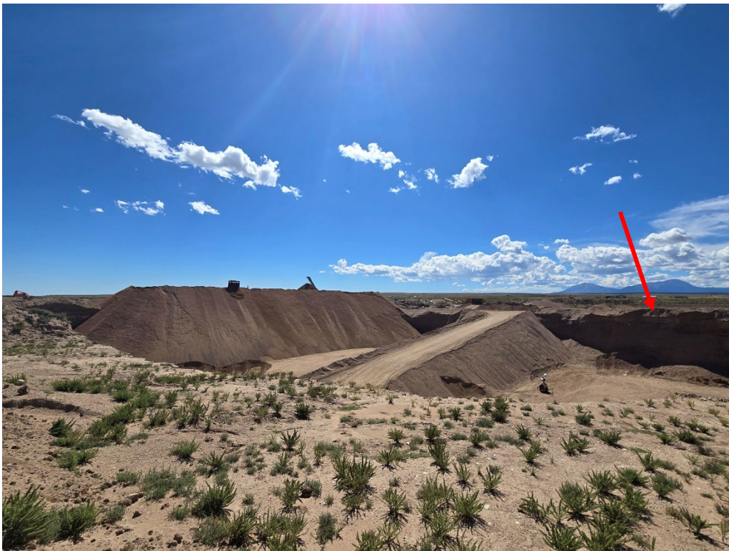
Photo 4: Looking southeast at the central pit. The arrow shows where the central pit and the west pit will be combined.
