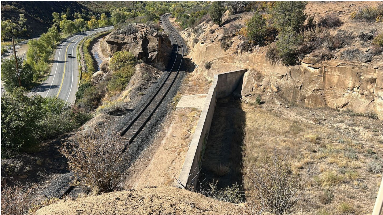
Figure 2: Pond E embankment and railroad
