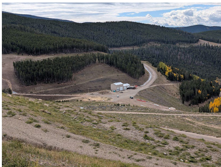
Slope above the Mine Shop has been regraded for stablization. A drainage channel and French drains were added.
