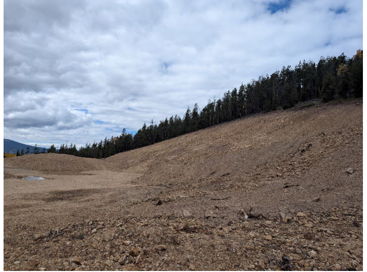
Sandstone Quarry slope has been regraded.
