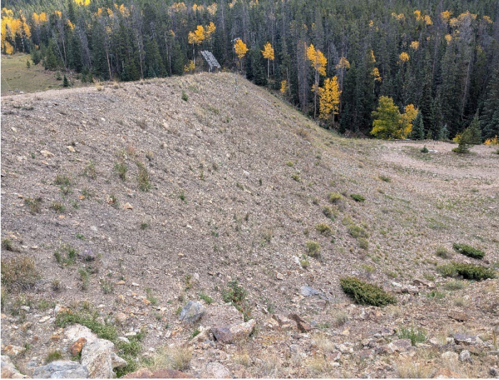
Sediment Pond dam appears stable. No seepage or stability concerns were observed.
