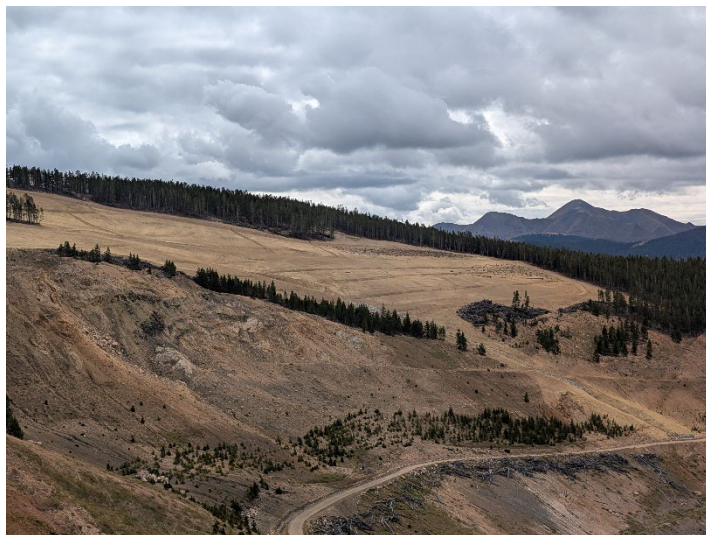
Land slide area above the North Pit has been logged and regraded with drainage features installed.
