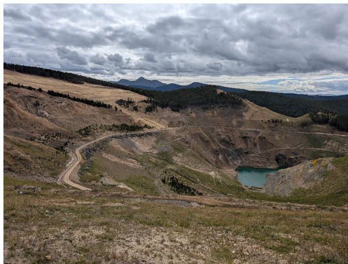
Landslide area above the North Pit viewed from the north side of the pit
