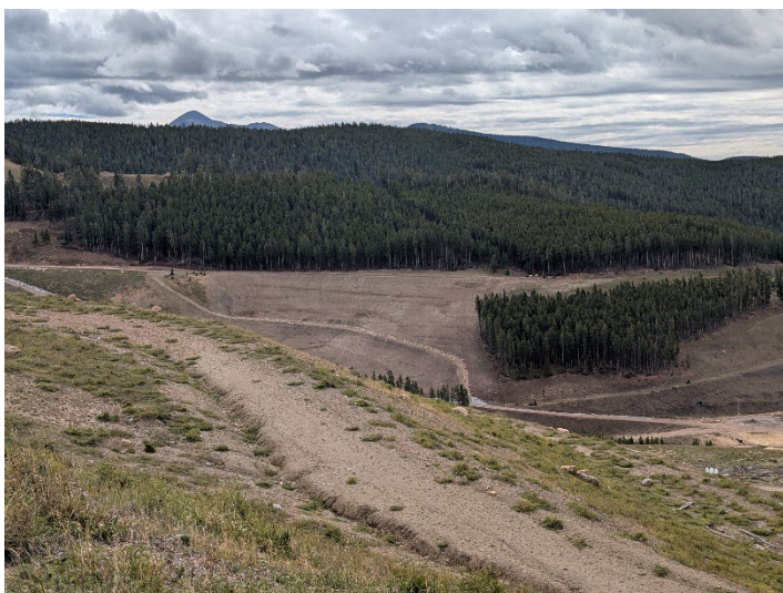
Slope above the Mine Shop has been regraded for stablization. A drainage channel and French drains were added.
