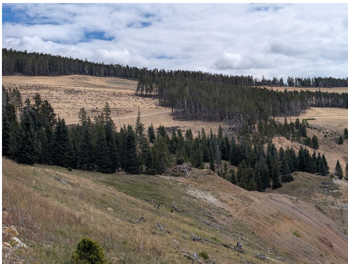
Land slide area above the North Pit has been logged and regraded with drainage features installed.
