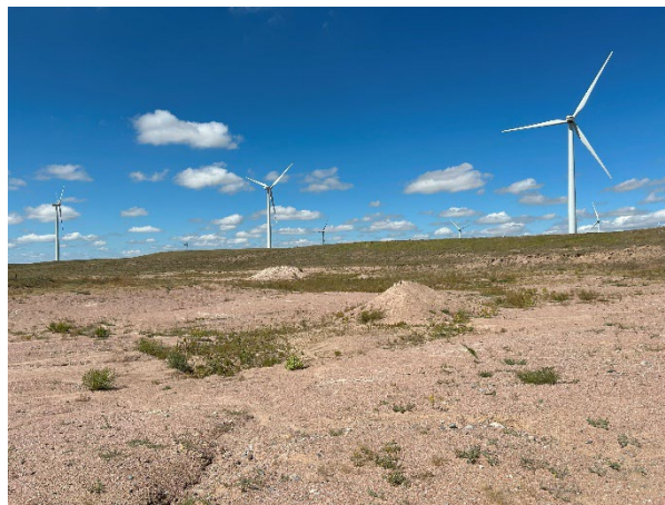
Photo 4: Primary pit floor, facing northwest.
