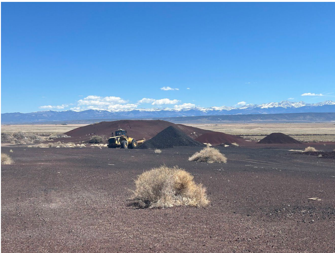
Photo 6: View of more stockpiled material and wheel loader, facing east.
