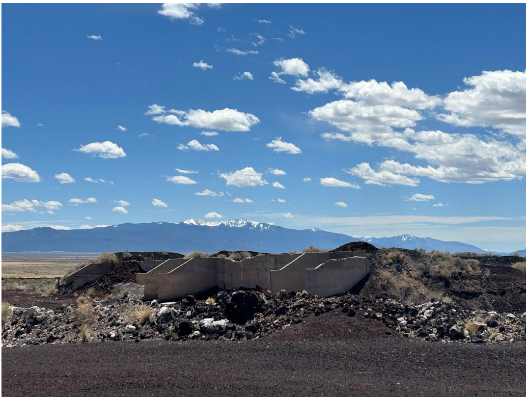
Photo 4: View of concrete containment bins nearby the concrete pad, facing south.
