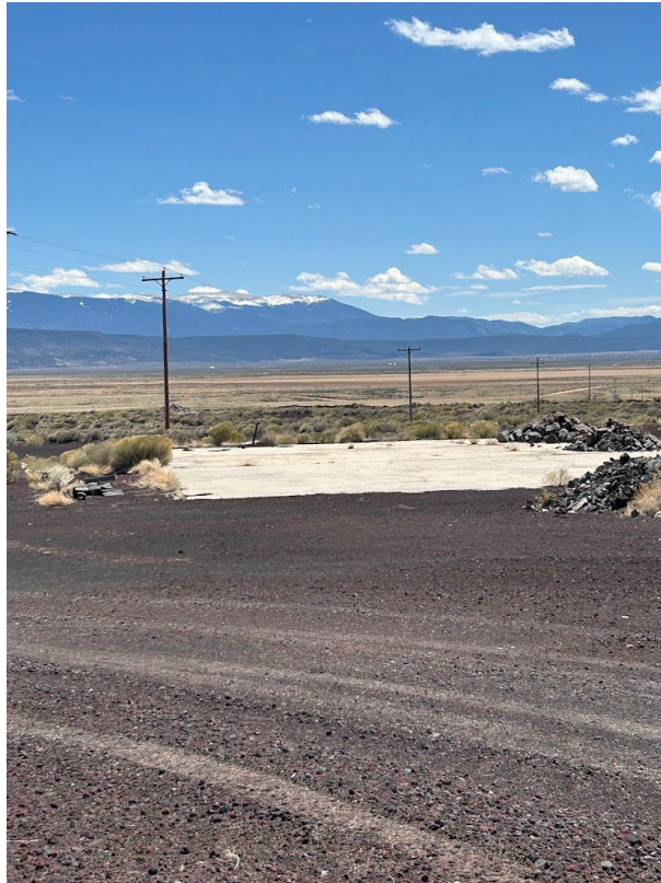
Photo 3: View of concrete slab with no equipment present, facing south.
