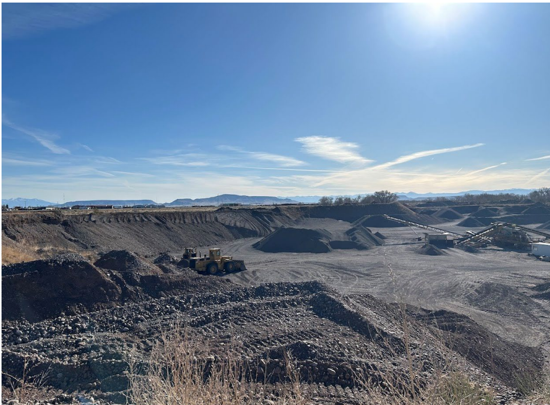
Photo 2: Primary working pit with material stockpiles and processing plant, facing northeast within the northern portion of the permit area.
