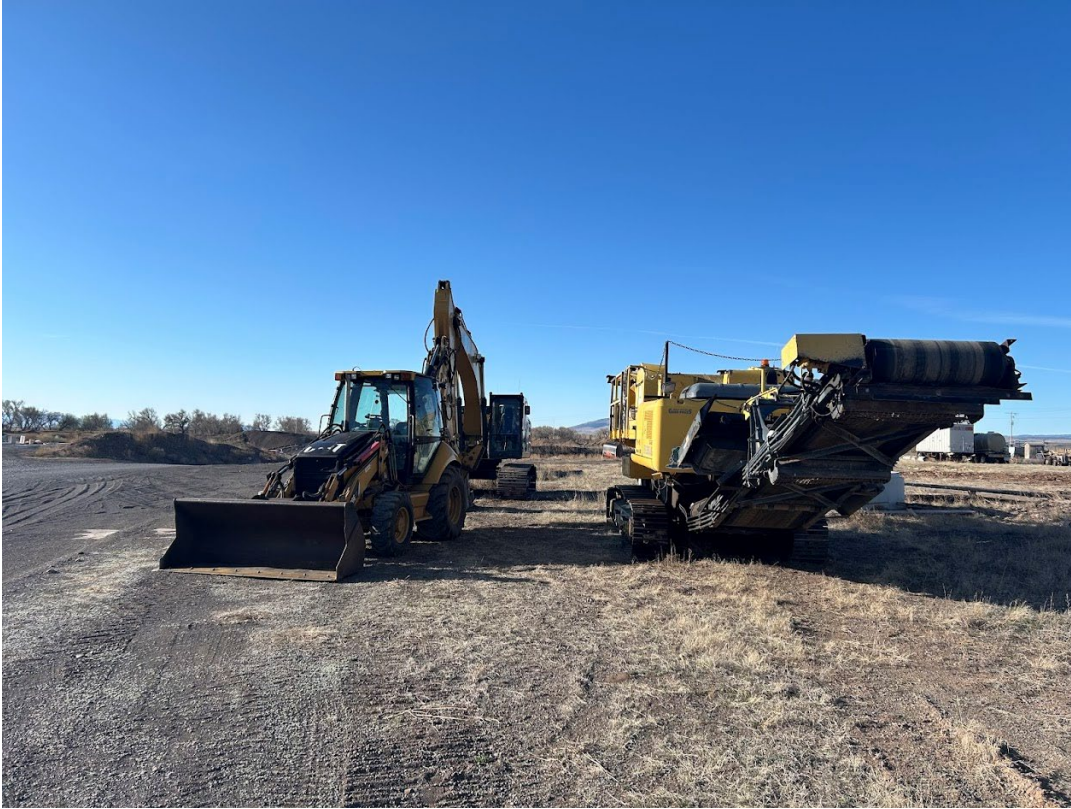
Photo 3: Mining equipment within laydown area adjacent to the southwest of the primary working pit, facing south.
