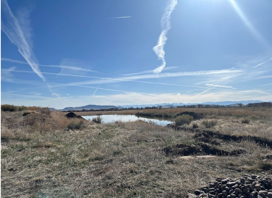
Photo 9: View of the groundwater recharge pond within the southwest corner of the AM-2 expansion area.
