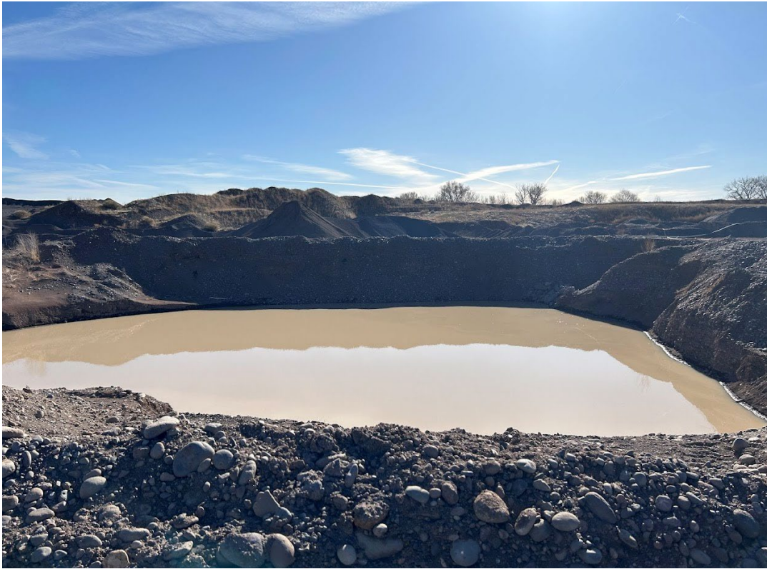
Photo 5: View of the sediment pond and clay embankments adjacent to the batch plant, facing east.
