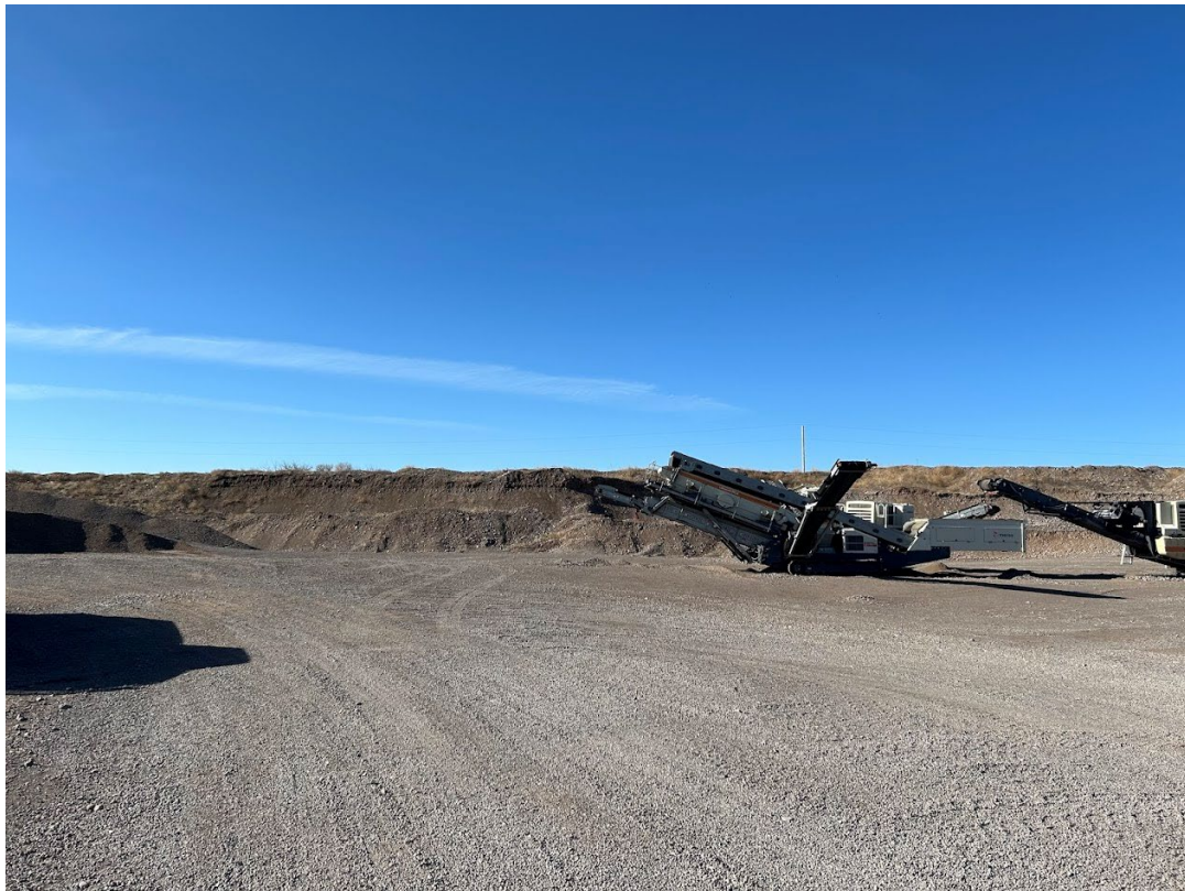
Photo 6: View of a stone crusher along the southern edge of the permit boundary, facing south. A vertical highwall exists along the southern permit boundary.
