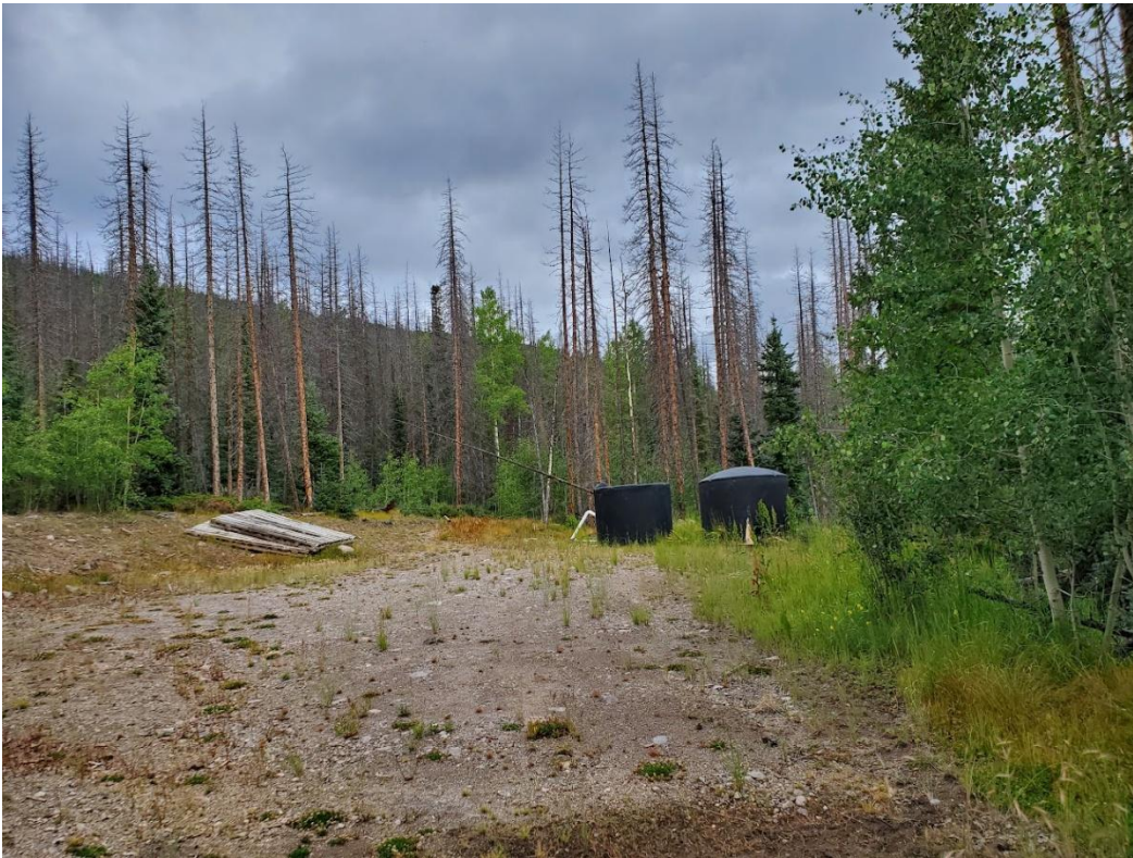
Photo 1: View to the north of pad with mud mats and empty water tanks.
