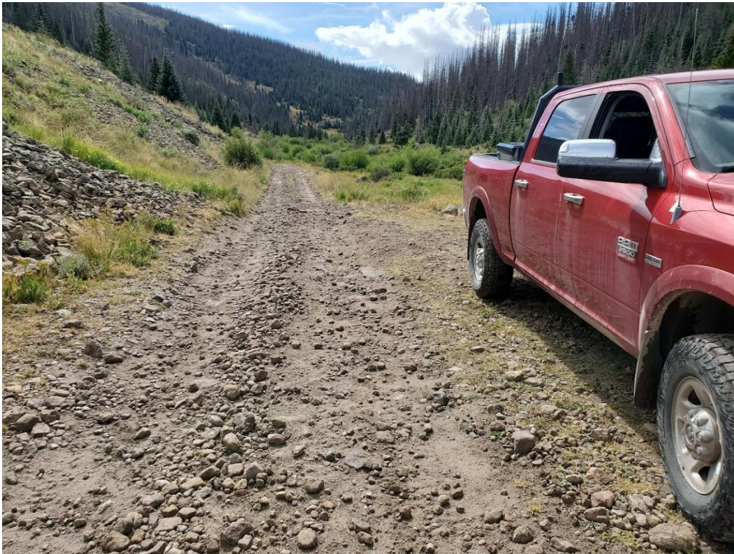
Photo 1: View to the south of the access road.
