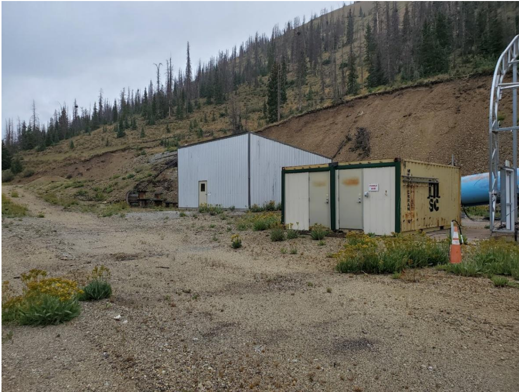
Photo 3: View to the northeast of the empty Fuel Storage Building.
