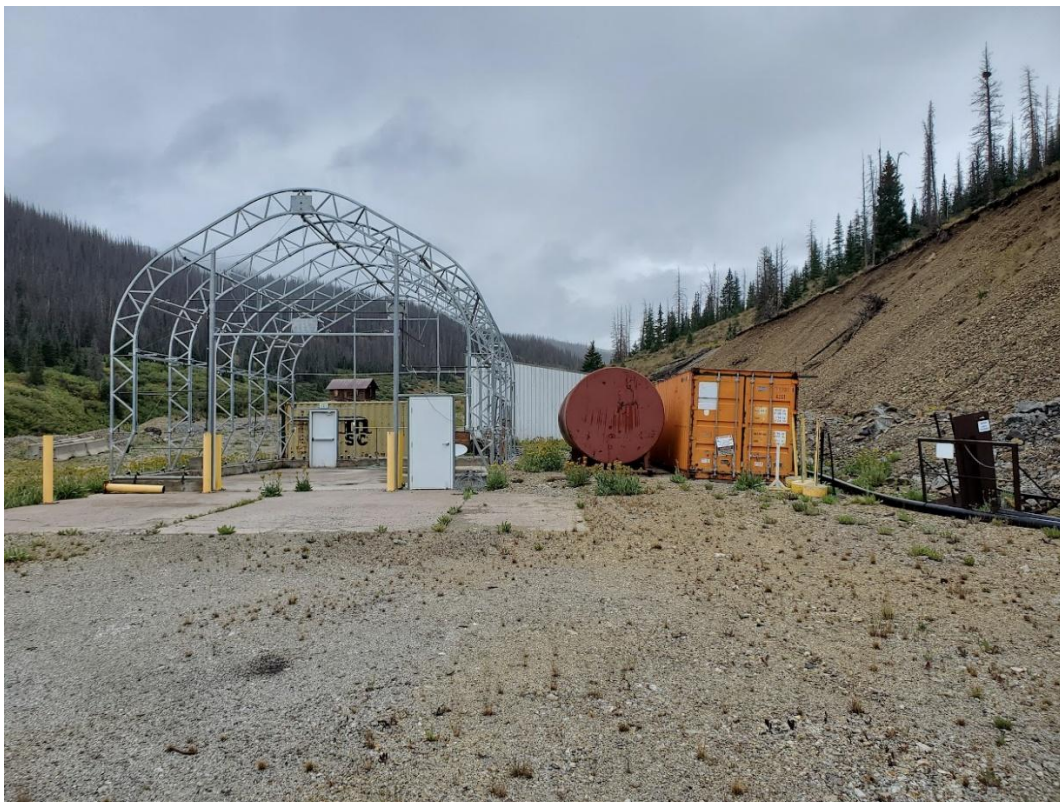
Photo 2: View to the north of maintenance shop skin, water tank, and Connex.
