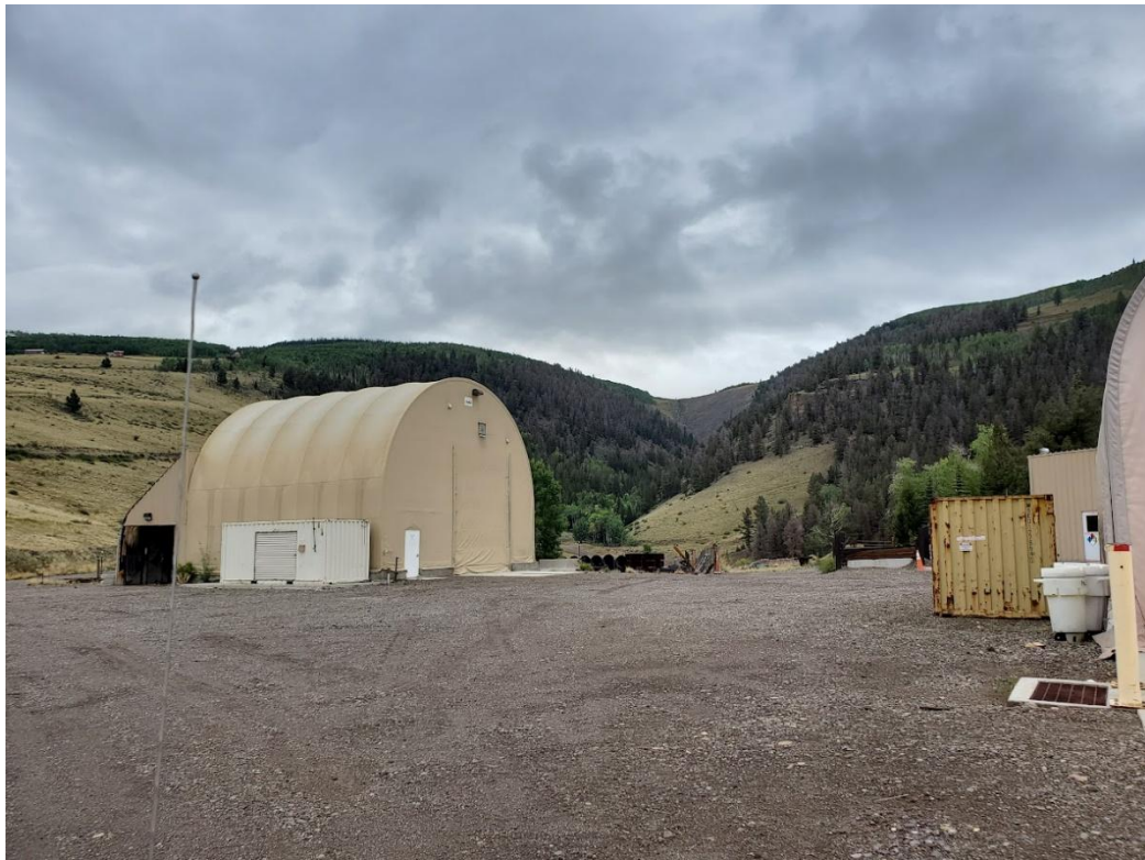
Photo 4: View to the northwest of facilities area.
