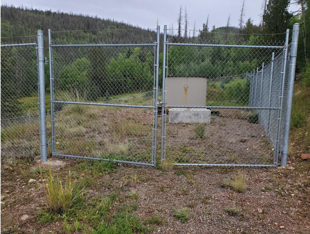
Photo 5: View to the northwest of Windy Gulch Vent Shaft
