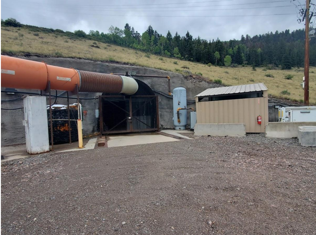
Photo 1: View to the west of 9400 Level Portal.
