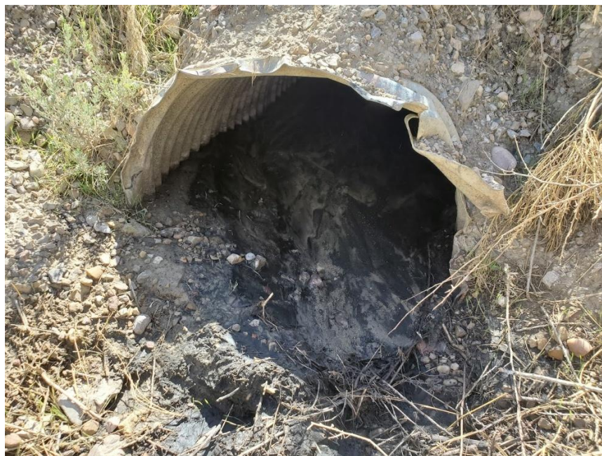
Photo 6: View to the south of the partially filled culvert above the SS-1 Pond.
