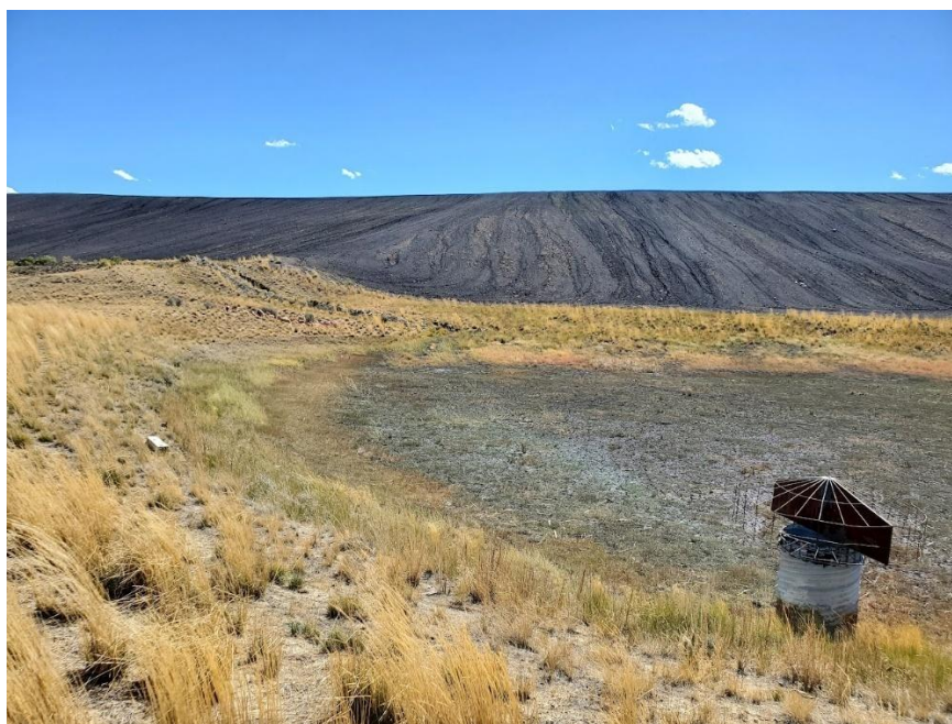
Photo 10: View to the south of the rills on the RP-2/3/4 Refuse Pile
