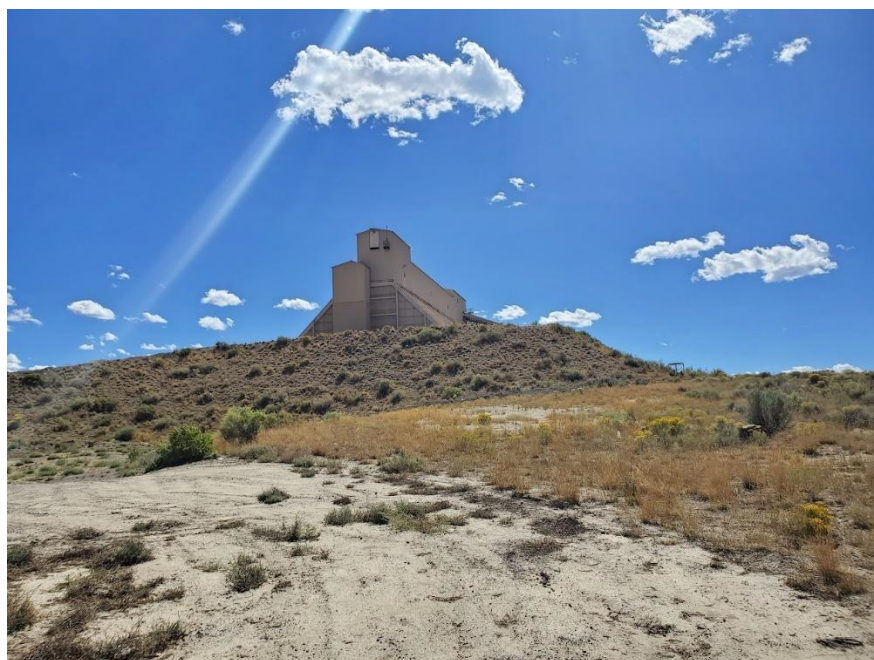
Photo 14: View to the south of the slopes below the Slot Storage Facility.
