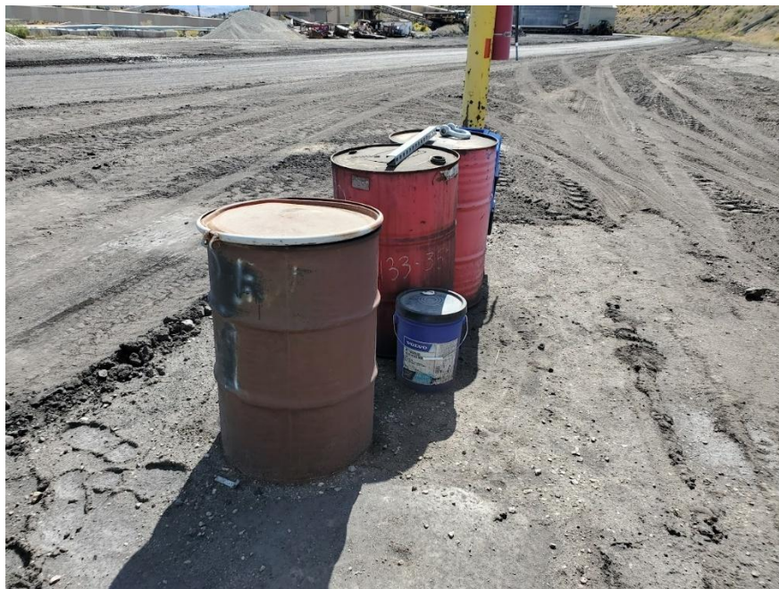
Photo 9: View to the southeast of barrels containing hydrocarbons outside of containment.
