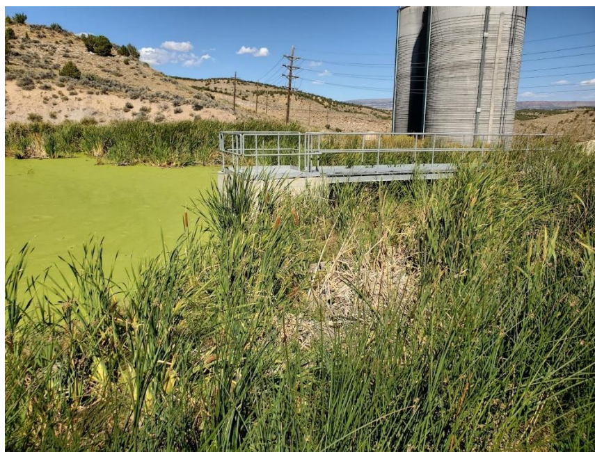
Photo 4: View to the west of outlet structure on PP-2 Pond.
