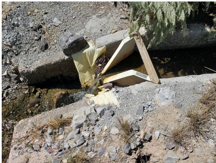
Photo 5: View to the south of the discharge at Last Chance Pond.
