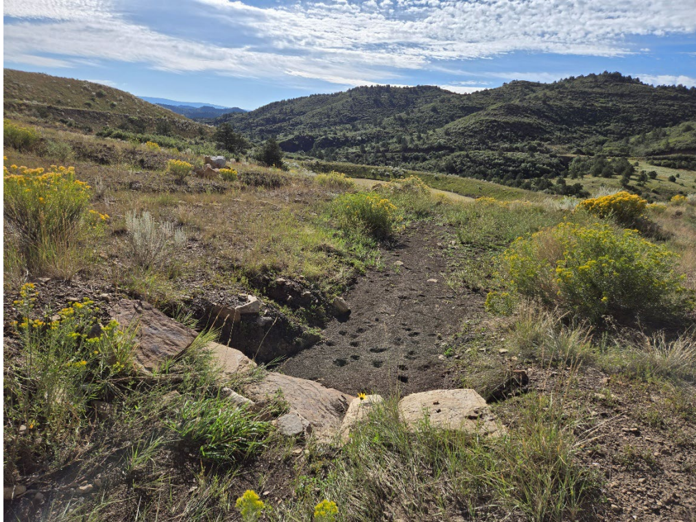
Photo 6: Full check-dams within ditch D8.
