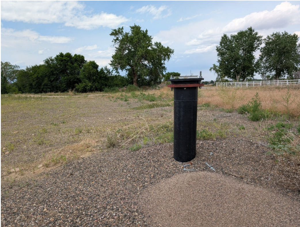
Photo 9: Looking at the standpipe for the Phase 1 French drain on the north end of the permit area. This end of the permit area has not been topsoiled or seeded.
