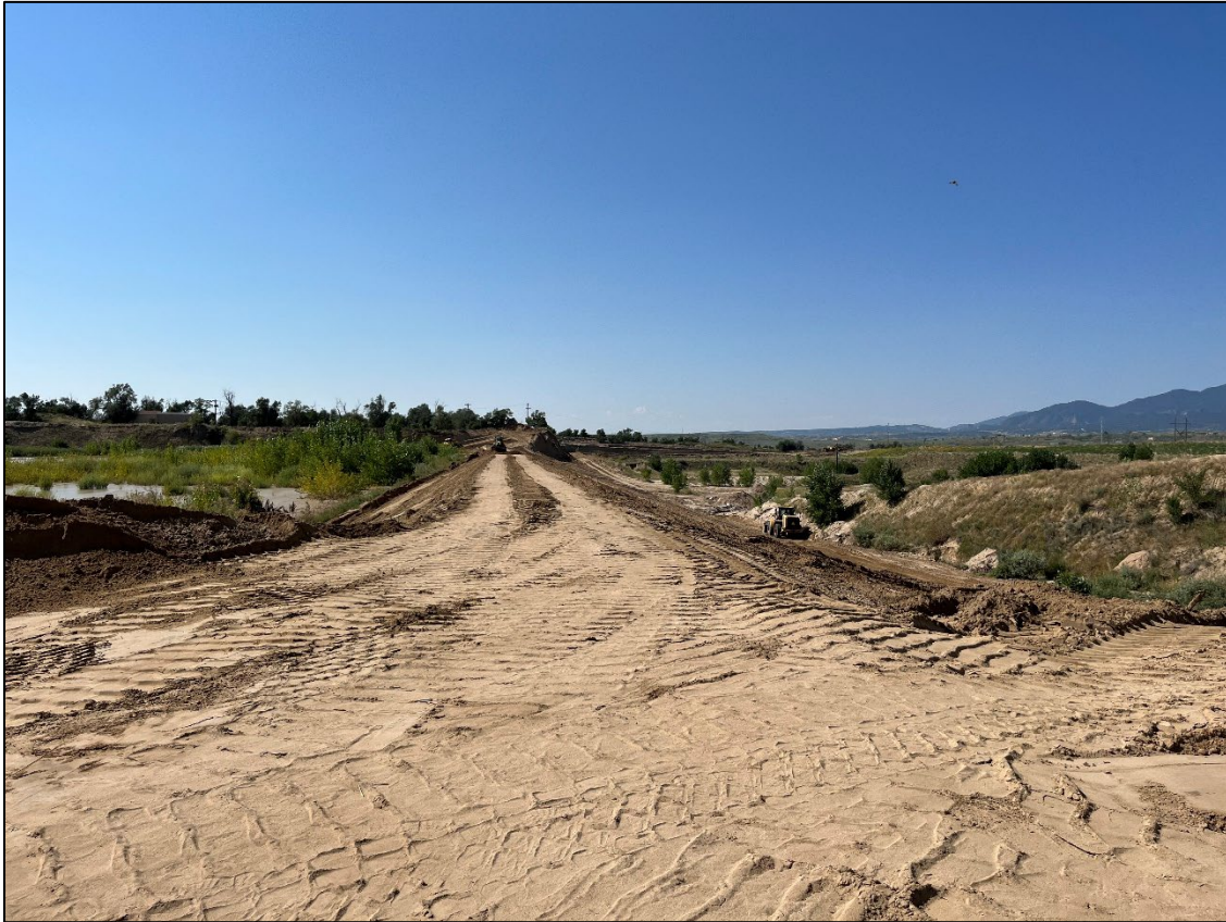
Photo 3: View south of the newly expanded berm on the west side of the wash pond.
