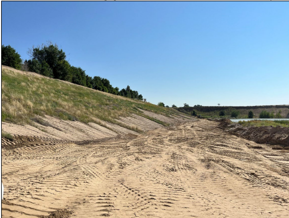
Photo 2: View east of the slope between Fountain Mutual Ditch and the easternmost large wash pond, recent repair of erosion is visible.
