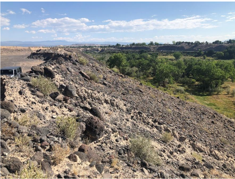
Berm and slope below the east pit area
