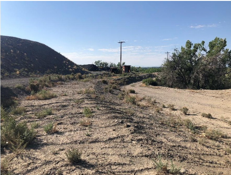
West side of affected area where a berm is needed
