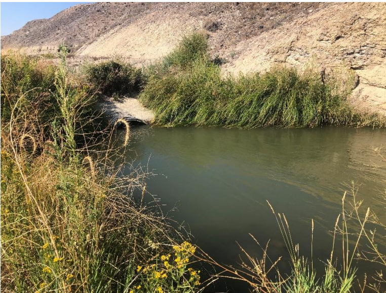
North Delta Canal on east side at transition from open channel to pipe
