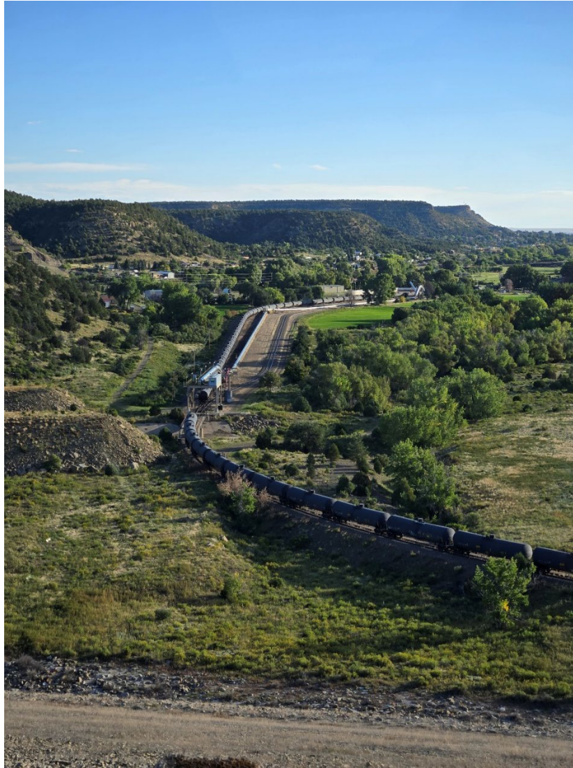
Photo 33: Jansen Loadout being utilized by a separate entity on the day of the inspection.
