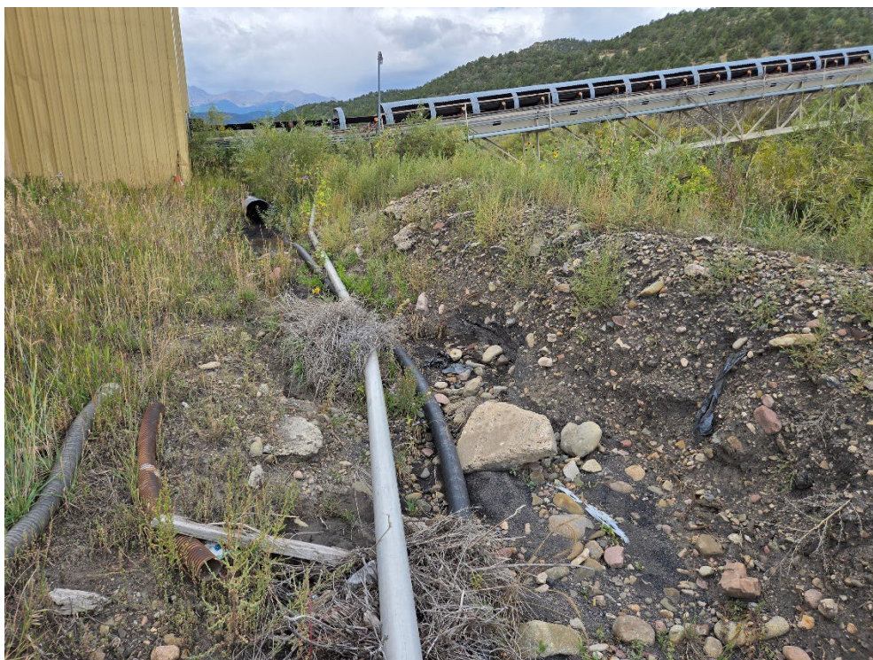
Photo 9: C64 outlet. South side of ditch D32A alongside showed minor signs of cutting, but the ditch appeared to be stable and no signs of erosion on the river side were observed.
