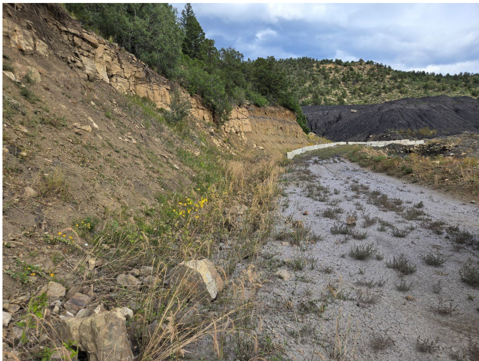
Photo 30: Looking north at the fine-grained grey material deposited on the road from ditch D56.
