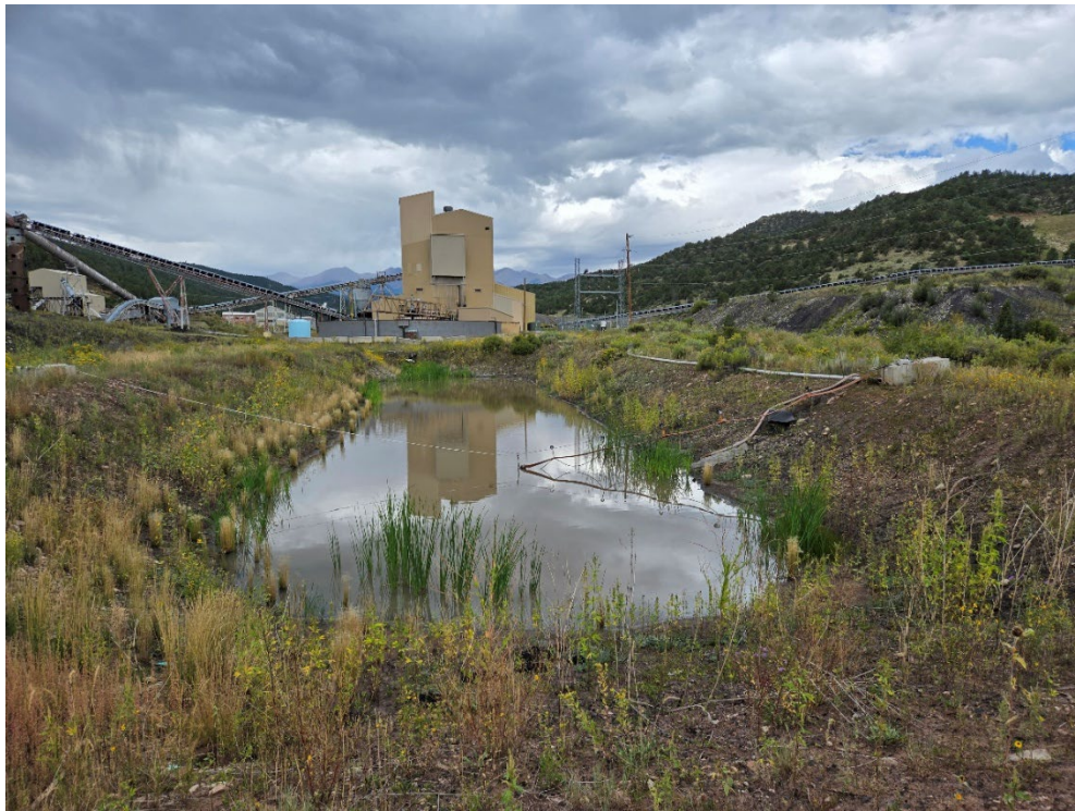
Photo 1: Looking west at Pond 006a.
