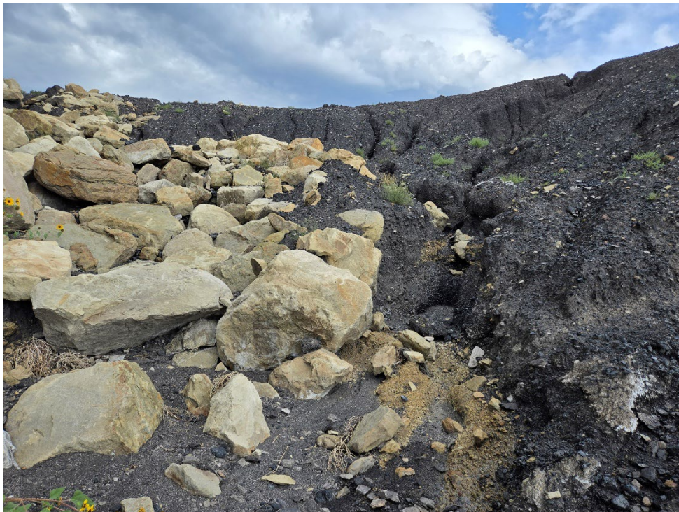
Photo 25: Looking up at the erosion gullies seen in Photo 24.
