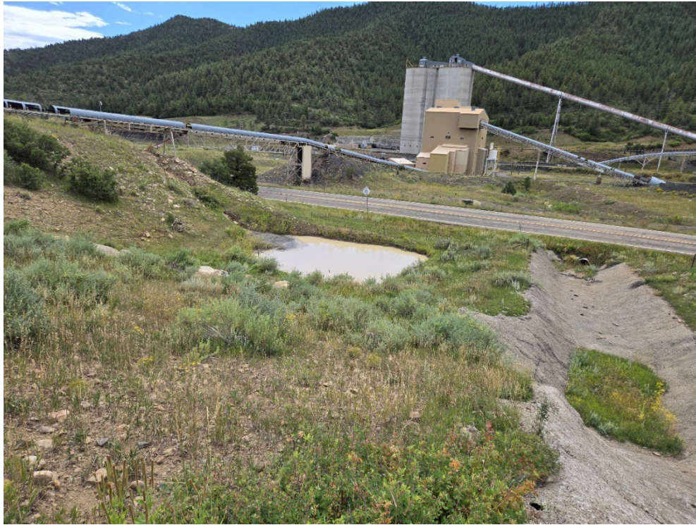
Photo 4: Looking south at Containment Area #5.
