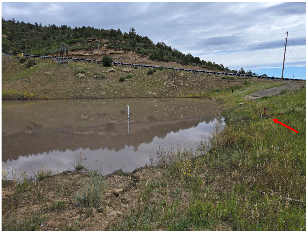
Photo 3: Looking east at the south bank of Pond 08. The arrow points to the principal spillway.
