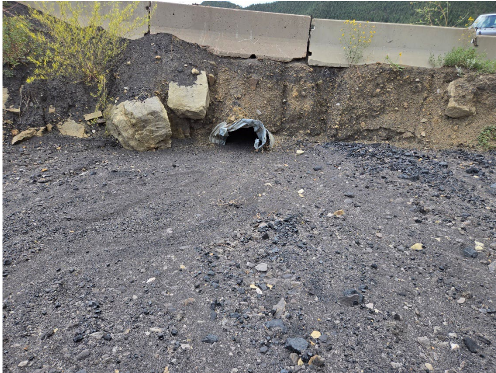
Photo 26: Looking south at the inlet side of C81.
