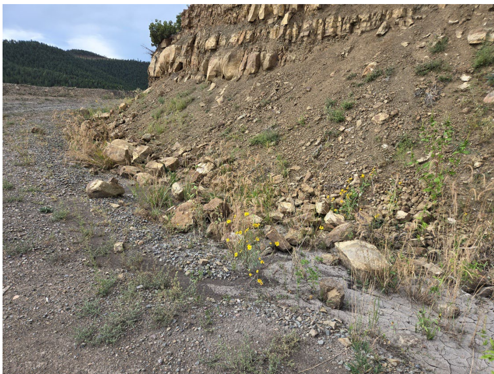
Photo 31: Looking southwest at the end of where sediment has accumulated within D56, near the bend in the haul road.
