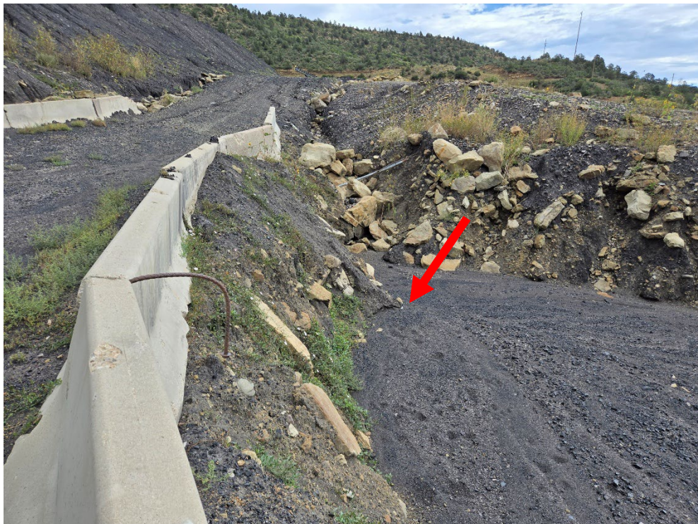
Photo 27: Looking east at the outlet side of C81 (buried).
