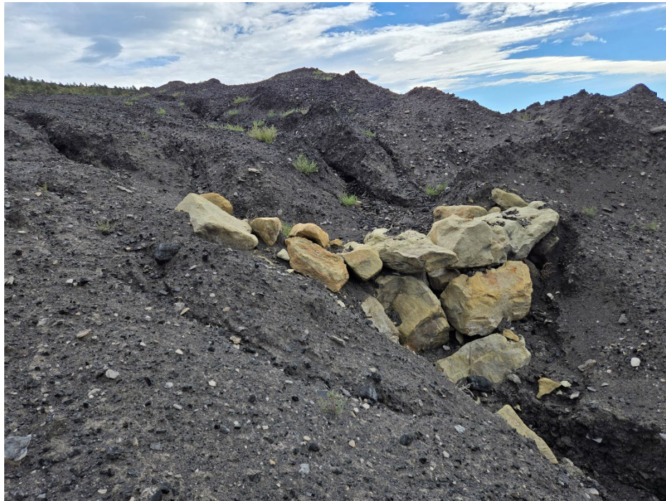
Photo 23: Looking at a check dam along the backside of the unreclaimed bench face, leading to the sediment basin.
