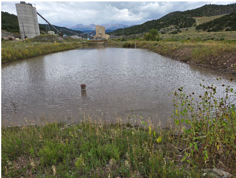
Photo 2: Looking west at Pond 007a.
