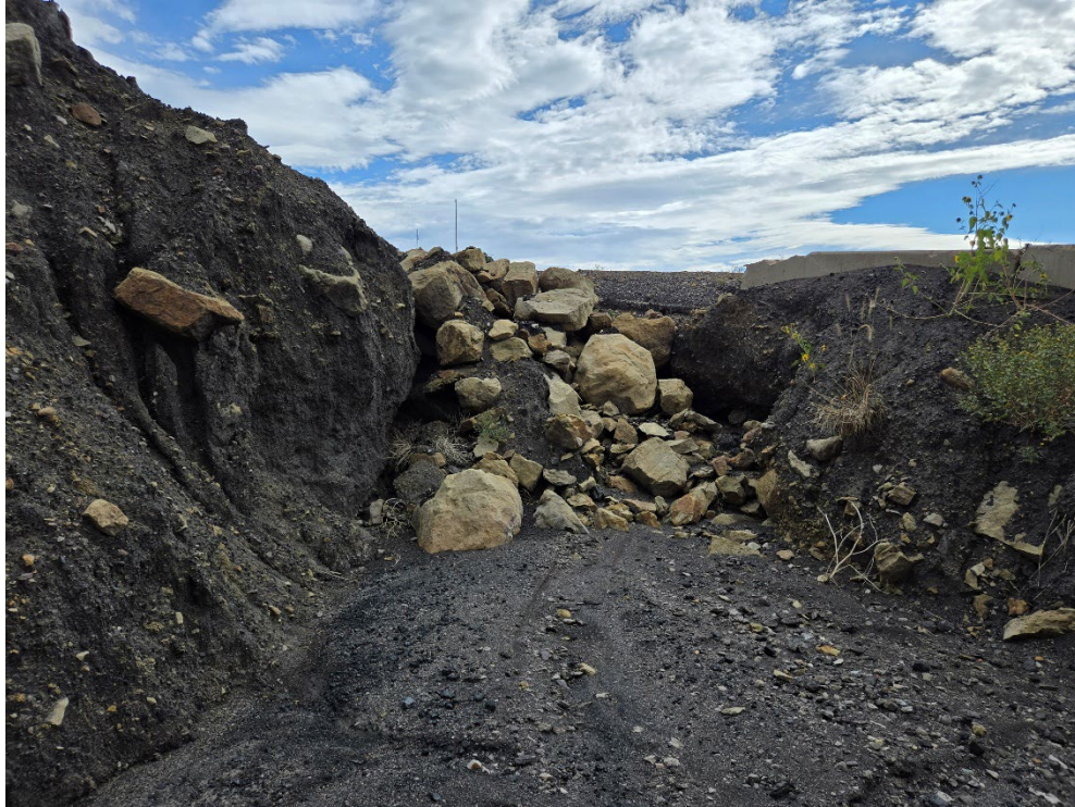
Photo 29: Looking east at the sediment deposited into the sediment basin on the north side of the road, by the ditches running along the north side of the road.
