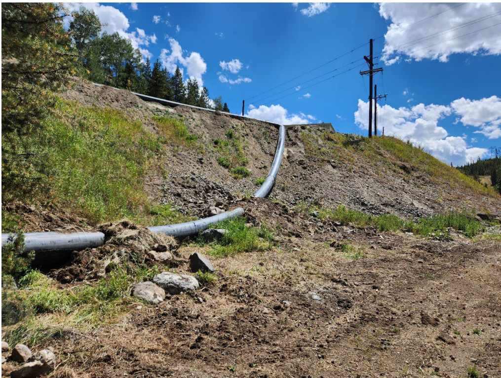
Photo 18. A 24-in leadoff pipe used to deposit tailings in the East Branch Trunk, looking south.
