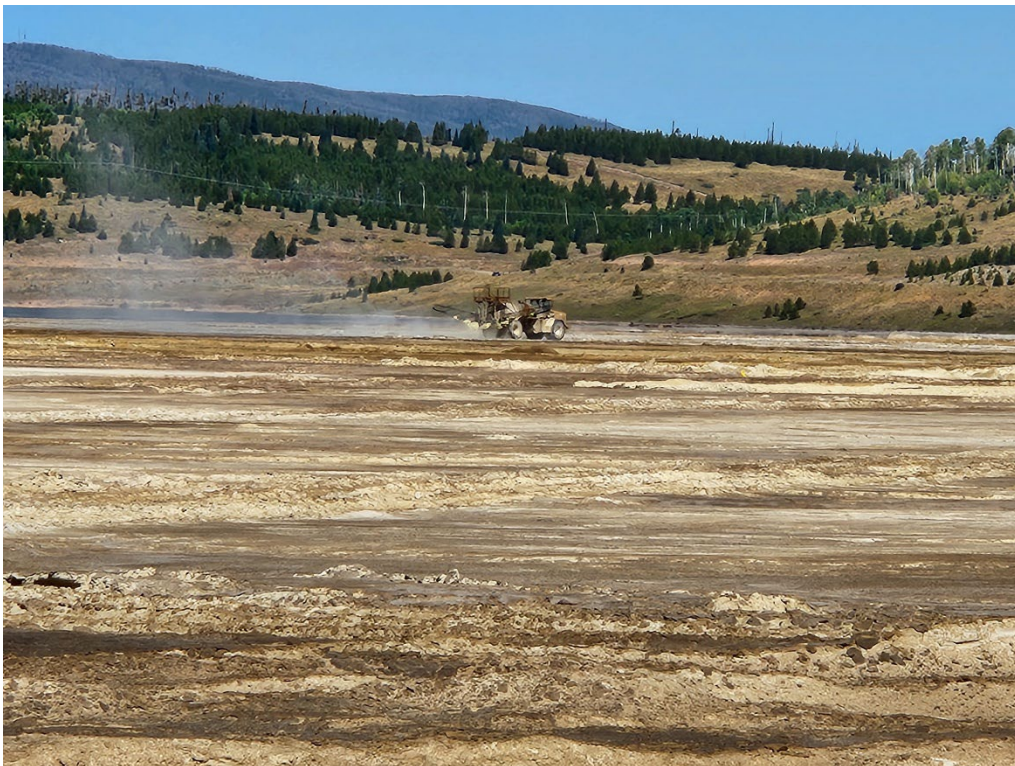
Photo 4. Equipment actively applying Coherex dust suppressant to the tailings.
