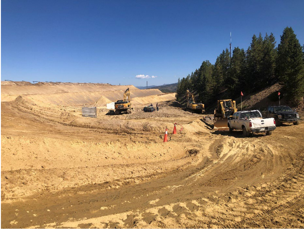
Photo 5. Construction area for the future seepage system return pipe.
