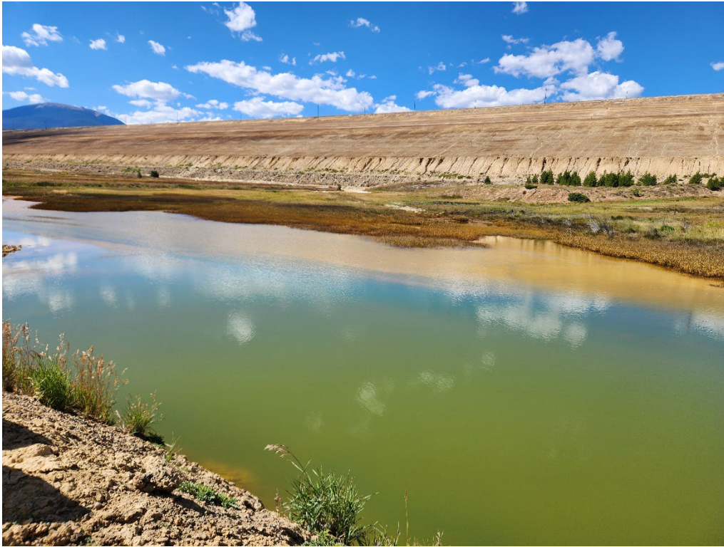
Photo 9. Seepage collection pond looking southeast.
