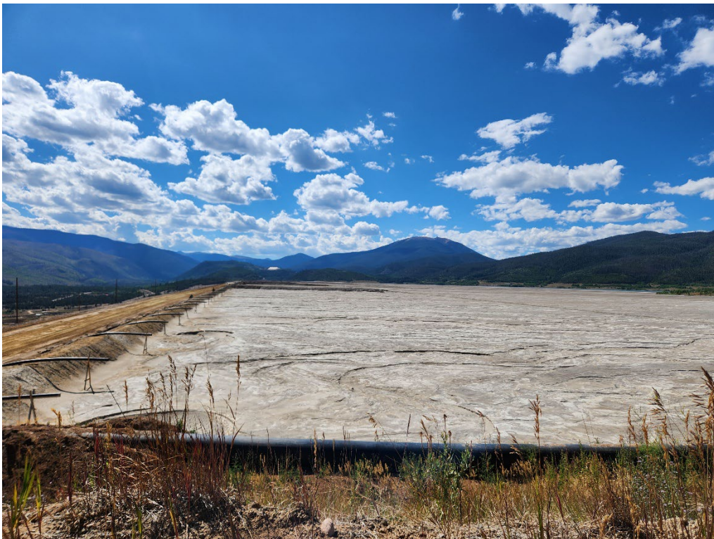
Photo 10. View of 1-Dam with Leadoff 9 in the foreground, looking southeast.
