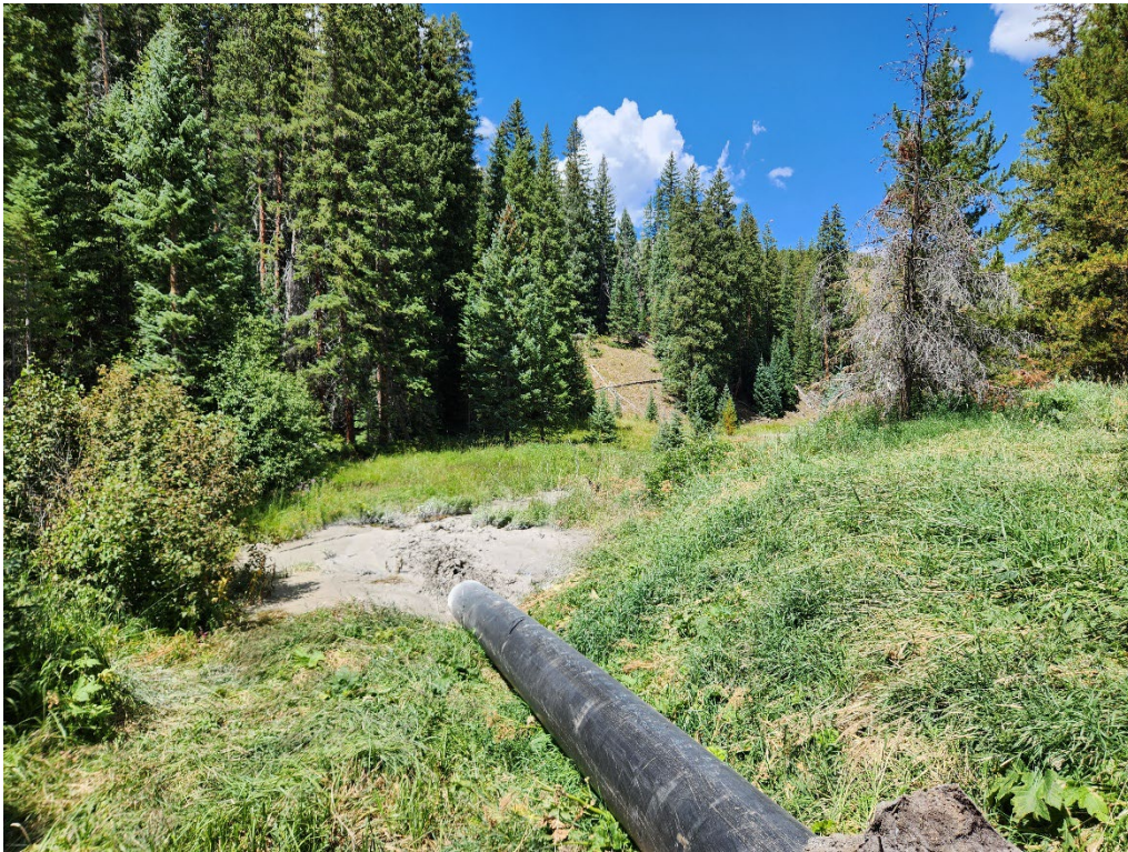
Photo 20. Tailings slurry flowing into the East Branch Trunk.
