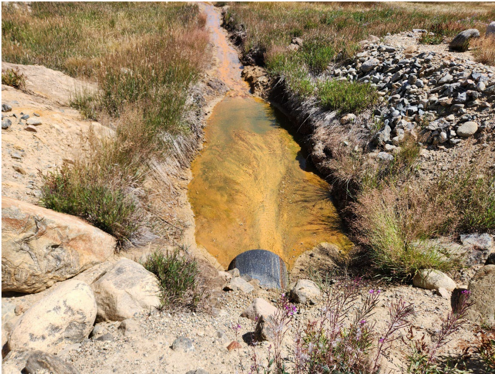
Photo 14. Culvert in the collection channel.
