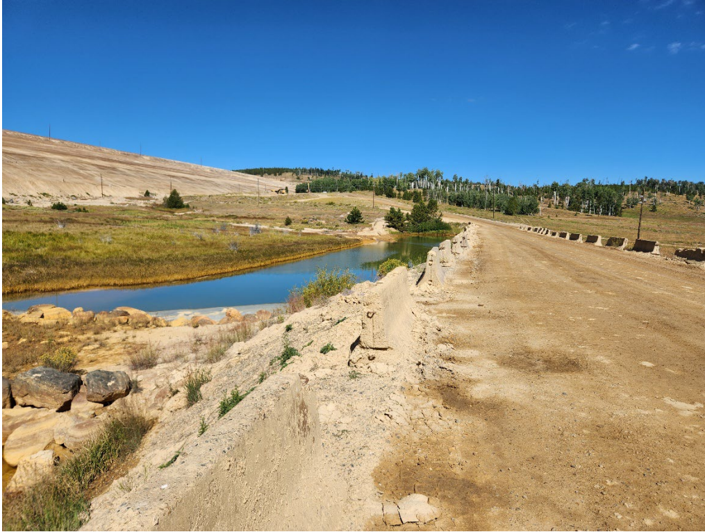
Photo 7. Seepage collection pond, looking northwest.
