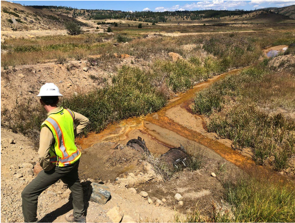
Photo 15. Abandoned decant lines below 1-Dam.
