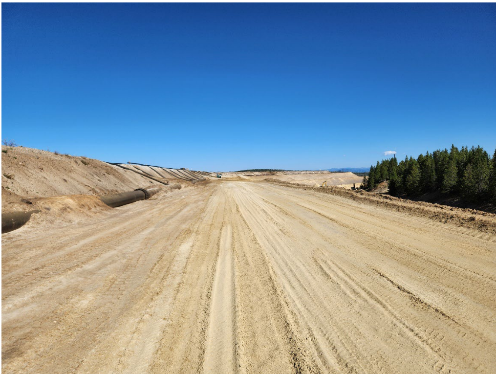
Photo 2. Access road that follows the tailing delivery line, looking northwest.
