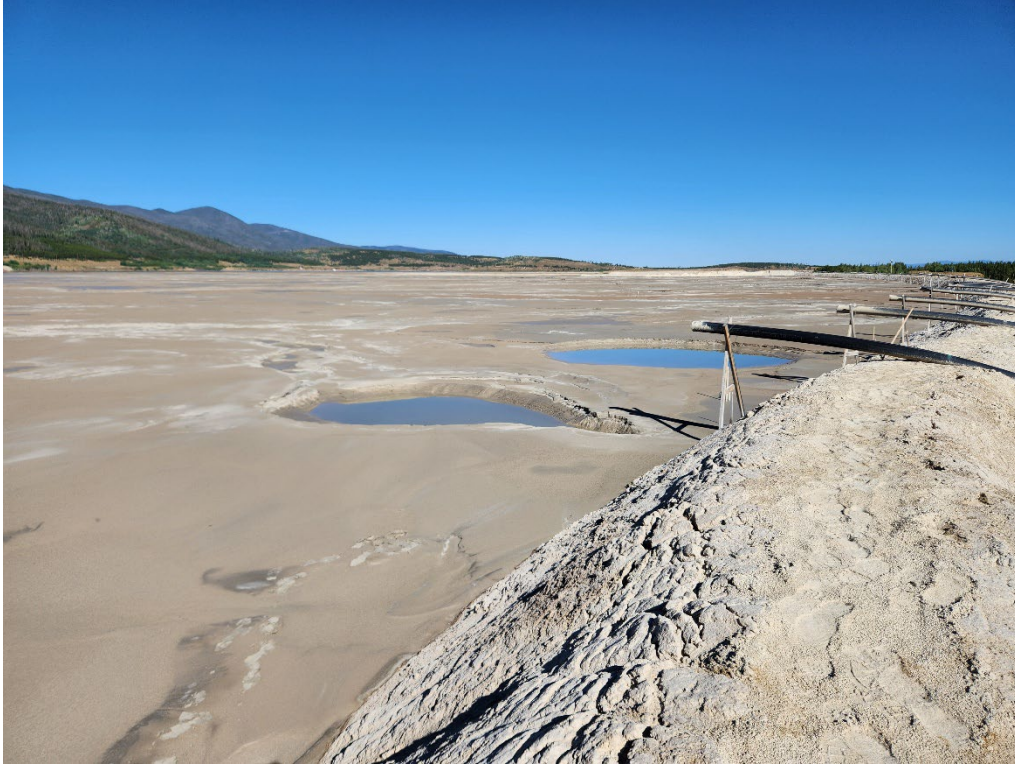
Photo 1. Spigots for 3-Dam, looking west.
