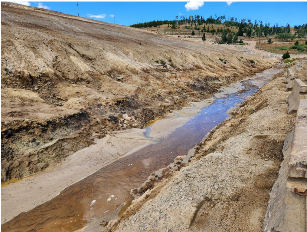
Photo 12. Horizontal drains below 1-Dam, looking north
