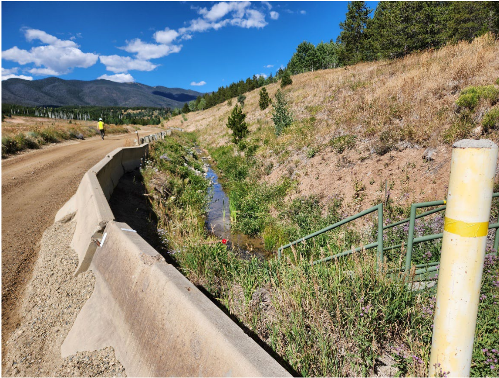
Photo 11. Ultimate Canal, looking west.
