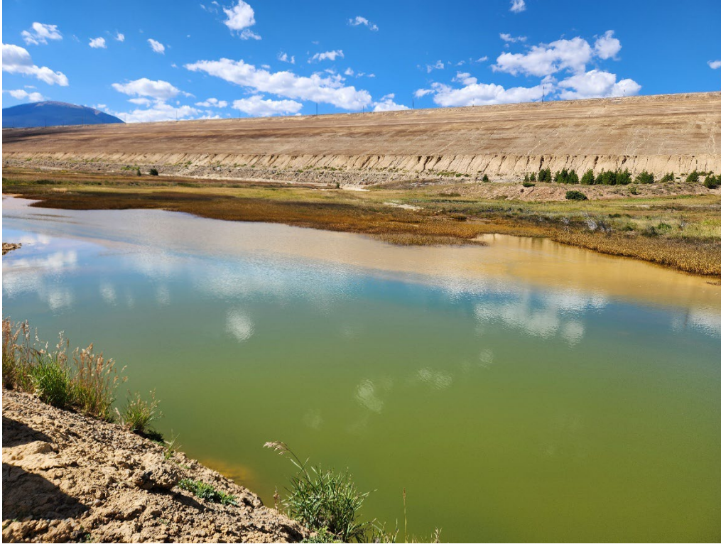
Photo 9. Seepage collection cell looking southeast.
