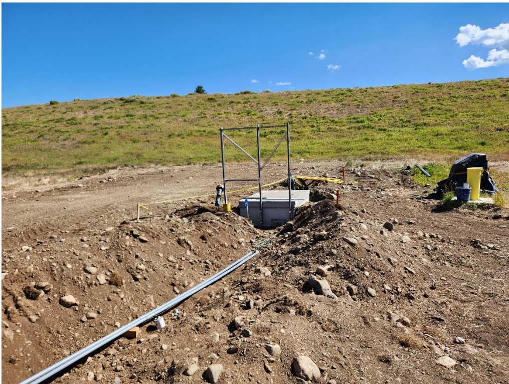
Photo 6. MLEX-6 Under construction.
