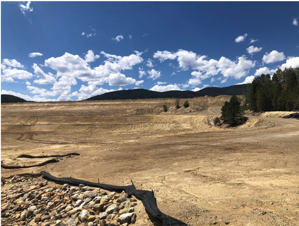
Photo 16. Buttress Phases 1 and 2 below 1-Dam.
