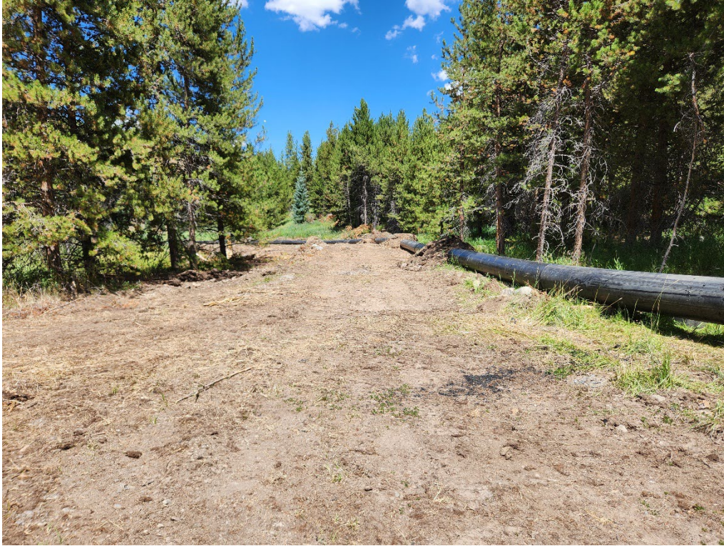
Photo 19. Road and pipeline leading down to the East Branch Trunk tailings deposit.
