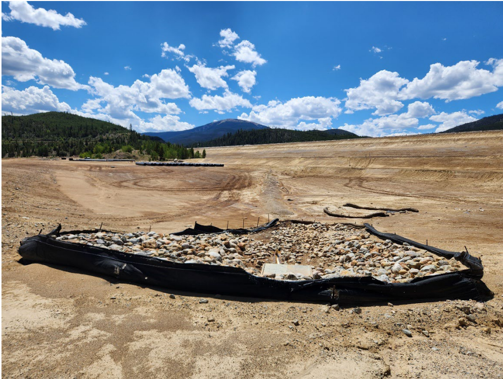
Photo 17. Buttress Phases 1 and 2 below 1-Dam, with seepage collection system above the north toe in foreground
