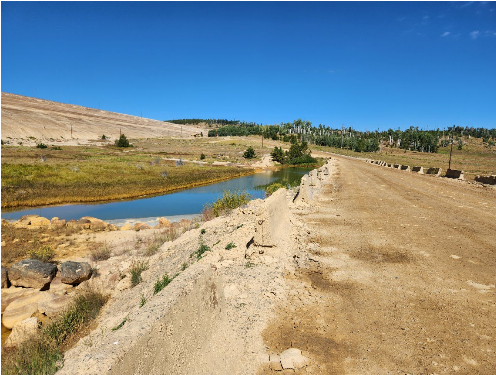
Photo 7. Seepage collection cell, looking northwest.
