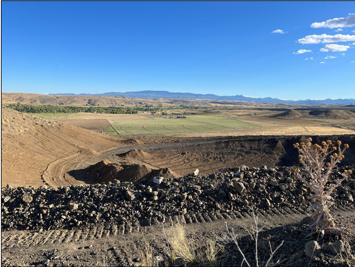
Photo 4: Continued view north into the pit area where several highwalls have been leveled to final grade.
