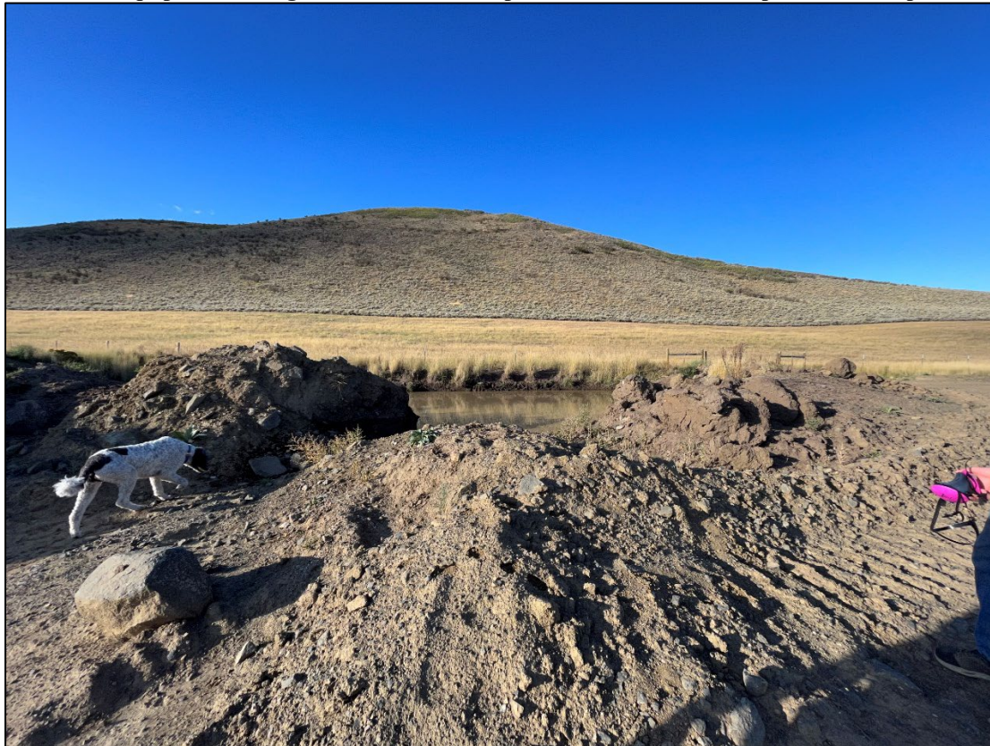
Photo 7: One of three small sediment sumps used to contain stormwater onsite.
