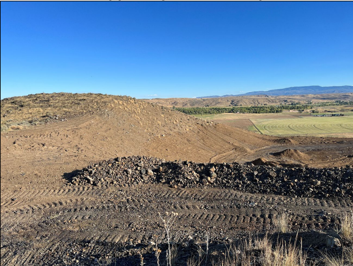
Photo 3: View north of the recently graded, topsoiled and seeded western end of the affected area.
