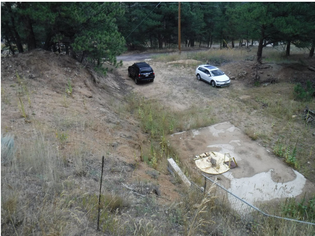
Photo 8: Area where the winch house and headframe were located
