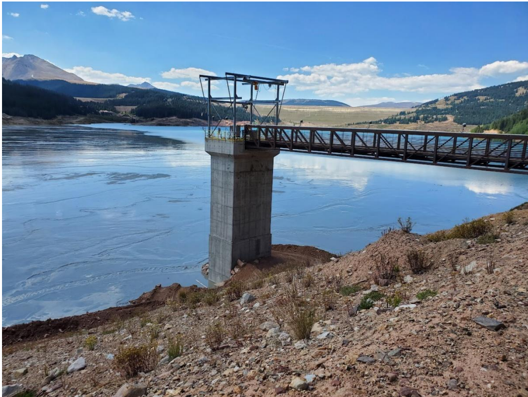
Photo 8: View to the southeast of Mayflower Tunnel
