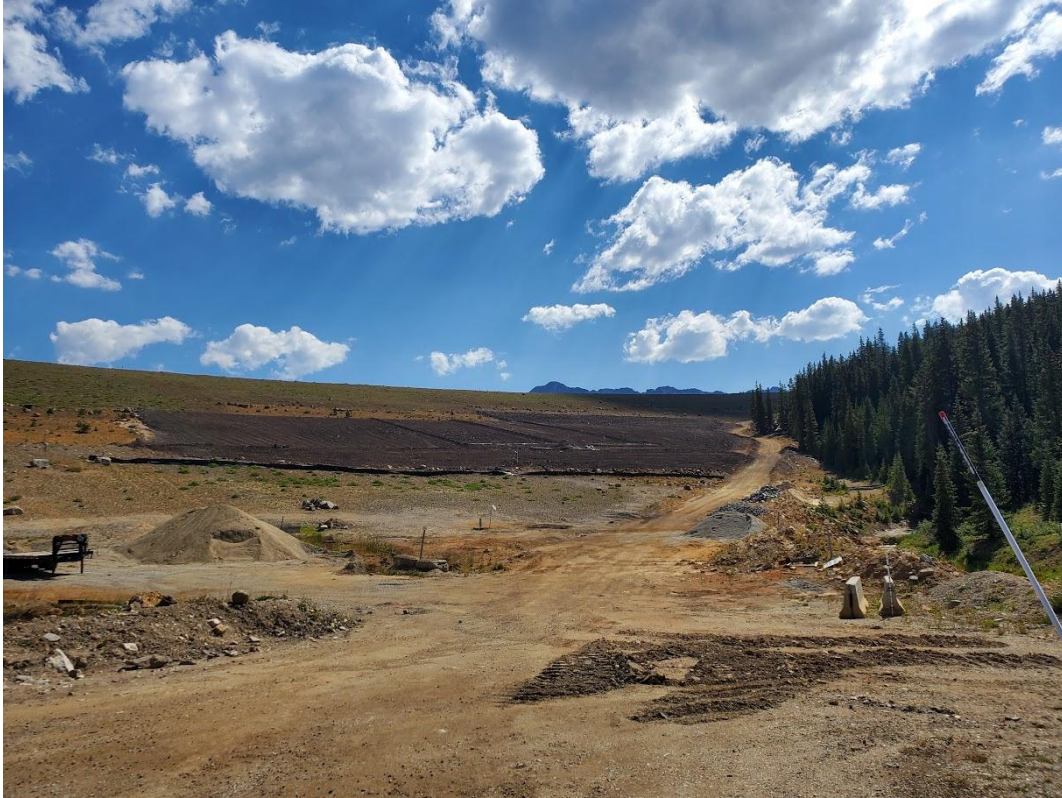
Photo 1: View to the east of the reclamation test plot on 1 Dam.
