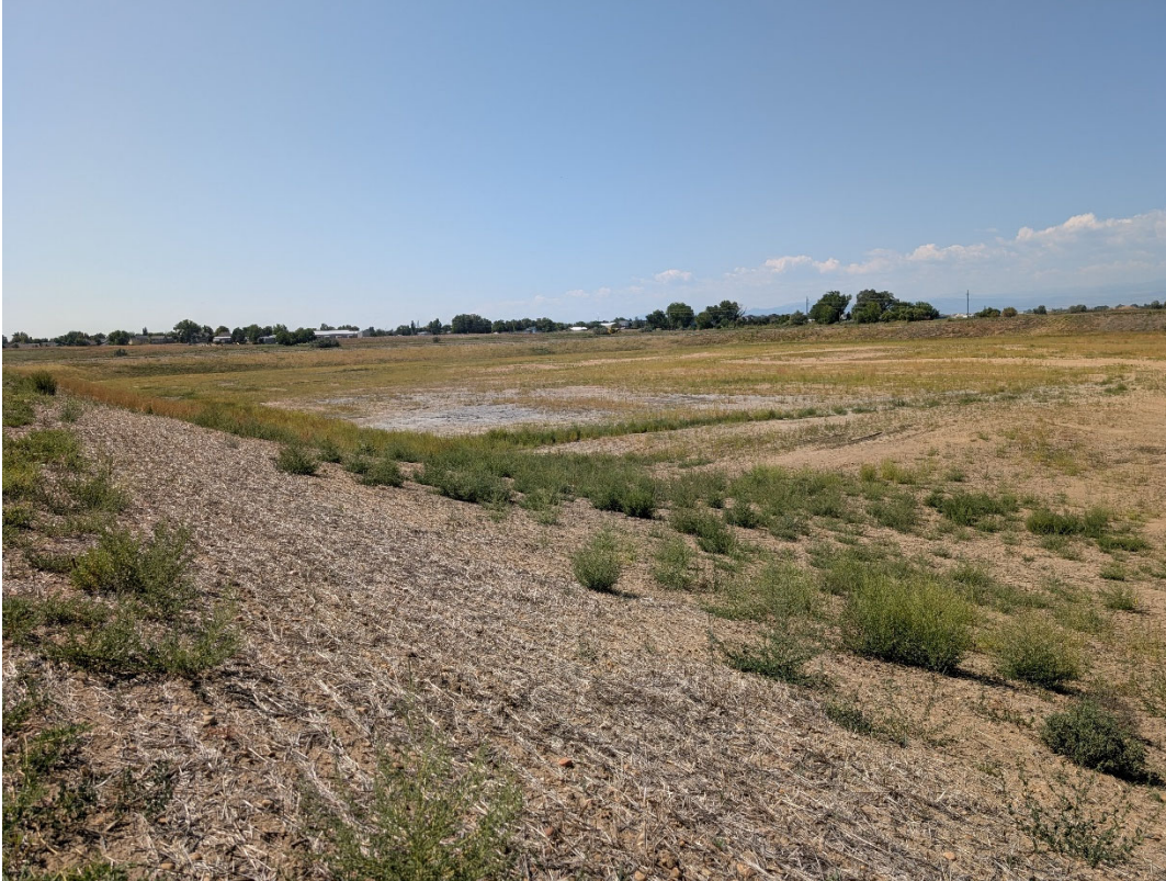
Photo 1: Looking southwest across the reservoir. Evidence of topsoiling, mulching and drill seeding observed on the slopes.
