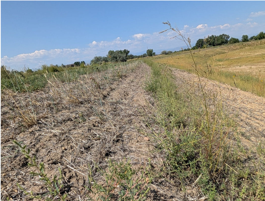
Photo 5: Closeup view of the topsoil placed above the water line on the south end of the reservoir.
