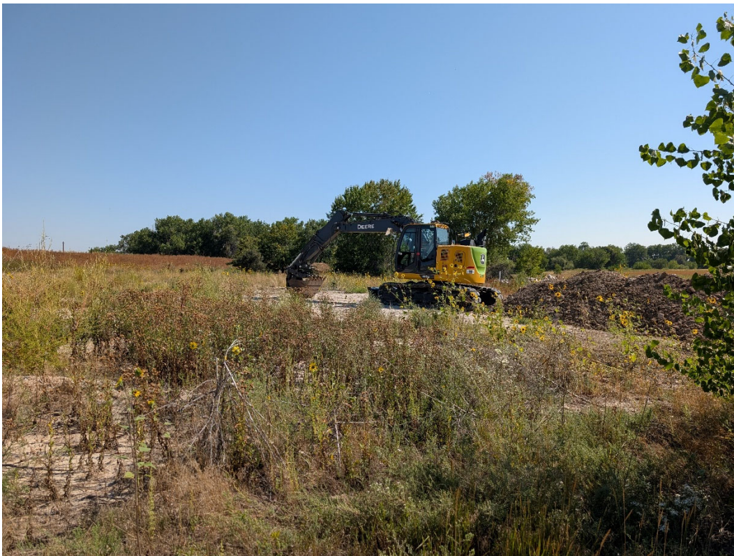
Photo 15: An excavator near the entrance next to some small stockpiles of material.
