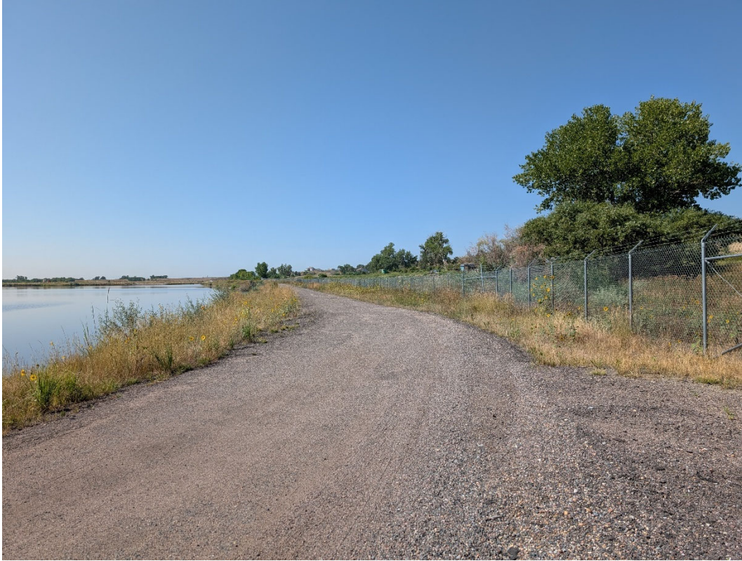
Photo 7: Looking south down the graveled access road adjacent to the south pond on the City of Thornton property.
