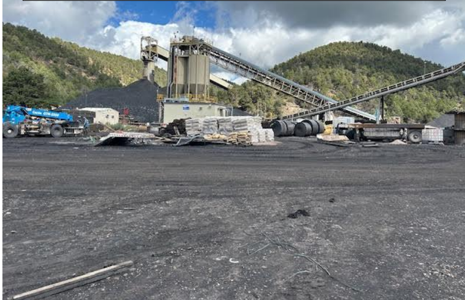
Photo 15: The laydown area north of the King II sediment pond.
